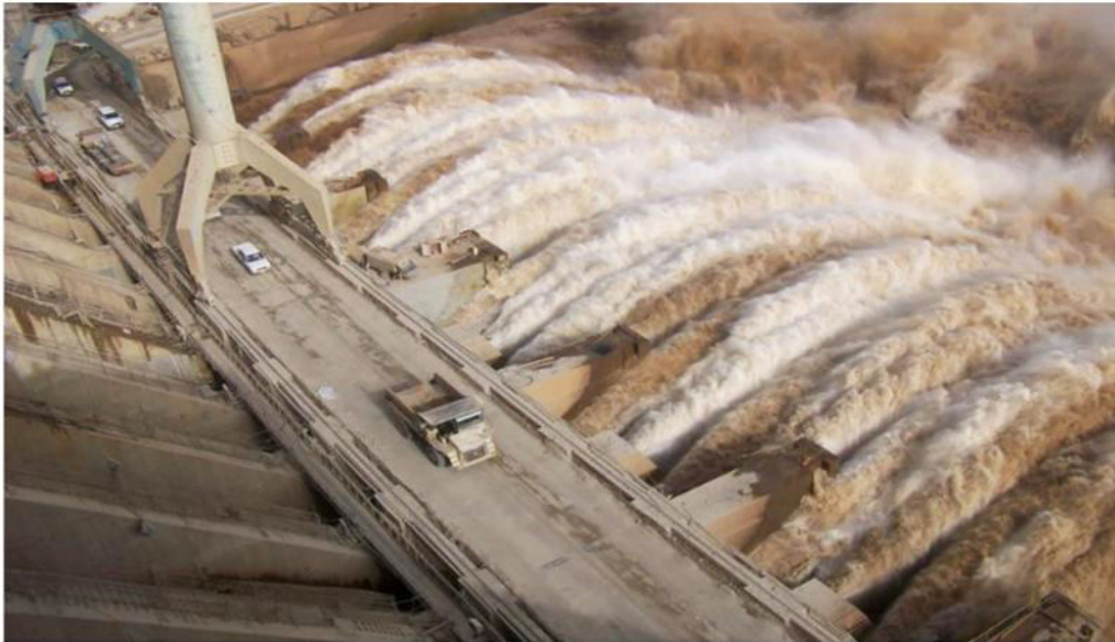
Merowe Dam and Hydropower plant Sudan
