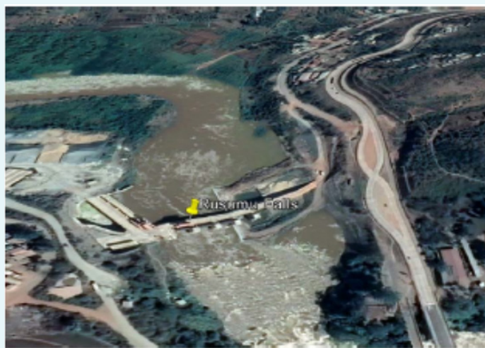
RUSUMO DAM. PICTURE FROM NELSAP ARCHIVE
