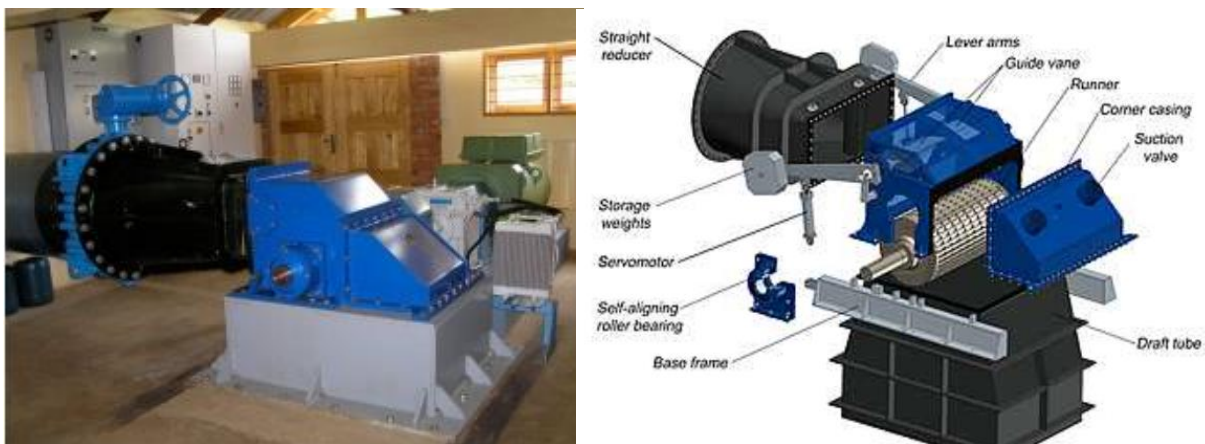
Figure 3-4: Installation of crossflow turbine at Kisiizi Hospital, Uganda (left). Schematic of Ossberger crossflow turbine (rights)
