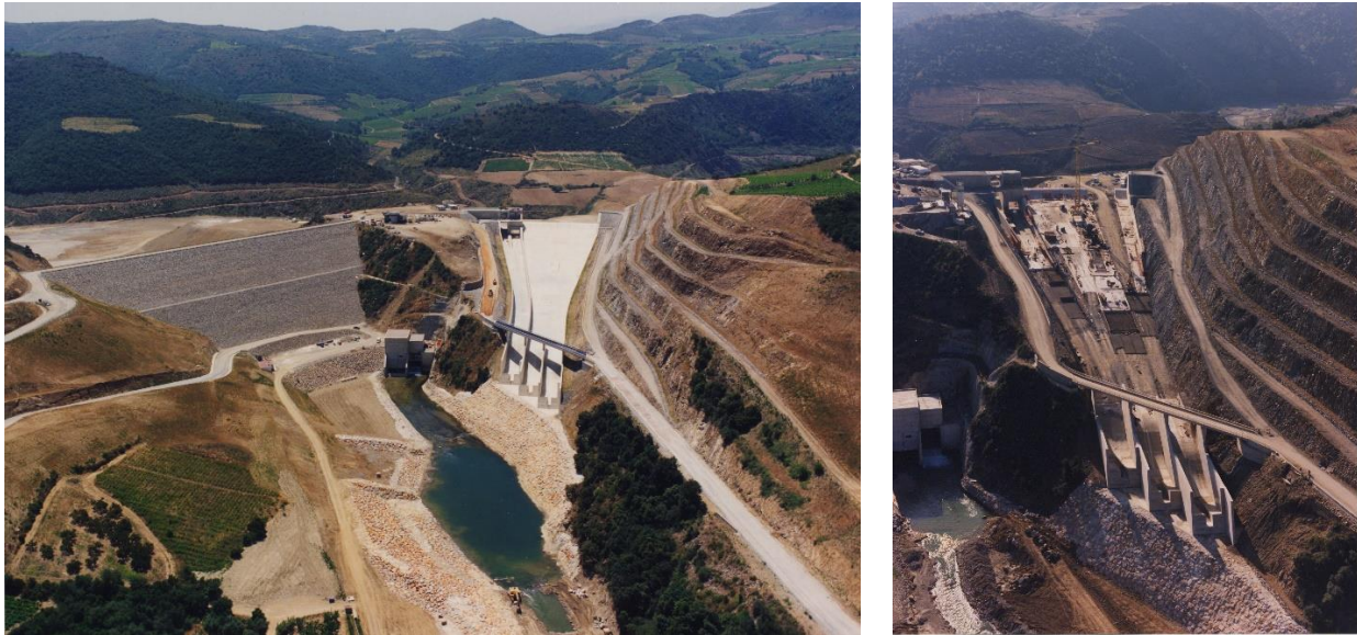
Figure 3-1: Agly dam during the construction (spillway on the right)
