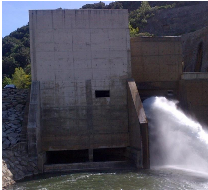
Figure 4-29: Hydropower plant, downstream view - compensation water through a fixed cone valve
