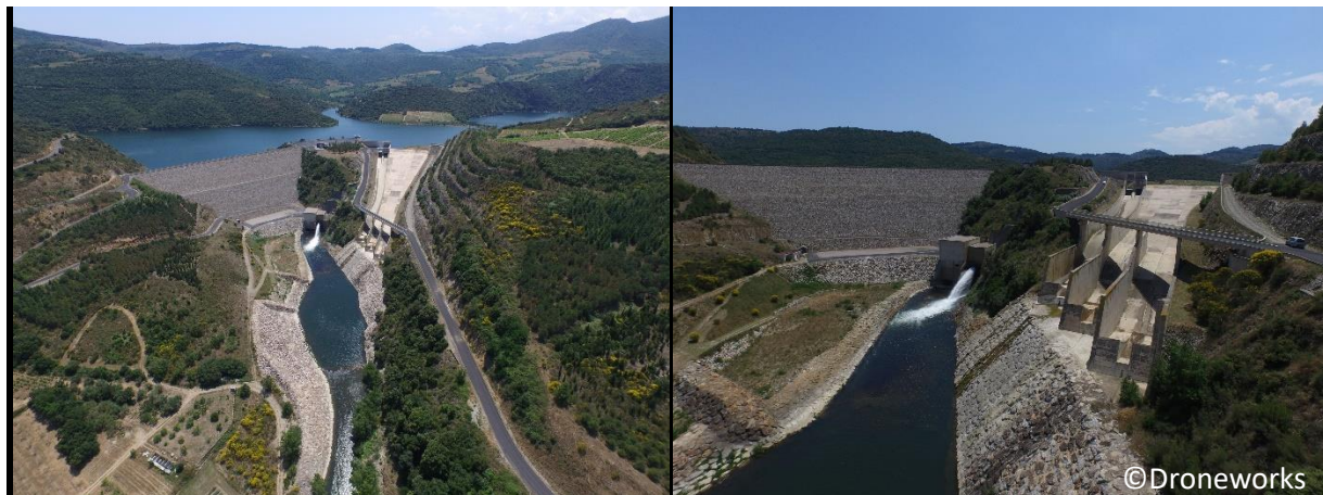
Figure 3-2: Agly dam recently
