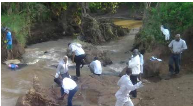
Examining damages in unmanaged watershed
