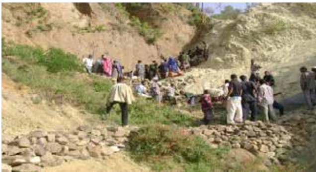
Community gully rehabilitation
