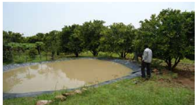
Rain water harvesting using geo membrane
