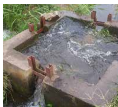
Water division box at secondary canal-Mubuku Irrigation Scheme
