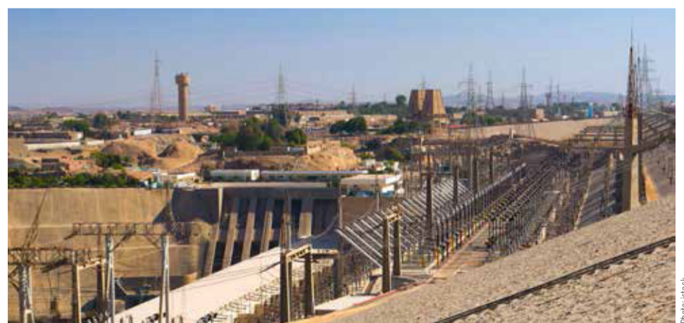
Hydroelectric power plant in Aswan dam (Egypt).
