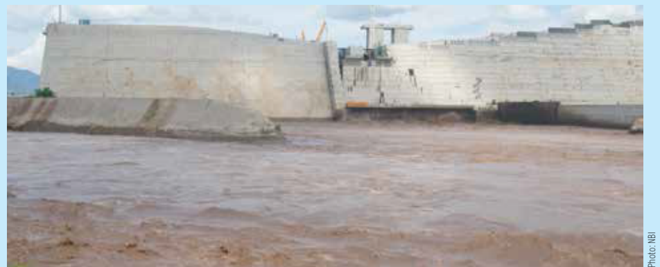
GERD dam under construction
