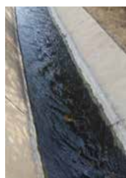
Main water division canal from river Sebwe-Mubuku Irrigation Scheme
