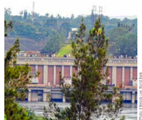
Kira power station Jinja, Uganda
