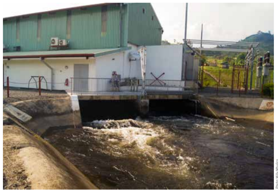
Troder Bugoye Hydropower plant in western Uganda
