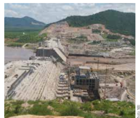
GERD dam under construction
