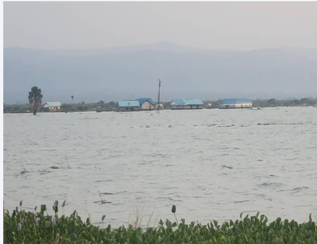
Butiaba Health Centre III still flooded and unusable (Photo taken in January 2022)
