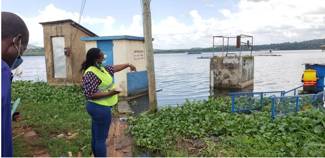
Existing Hydromet station
