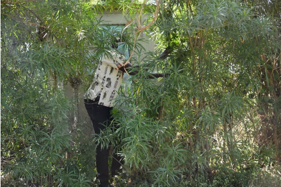
Accessing the concrete structure at the station
