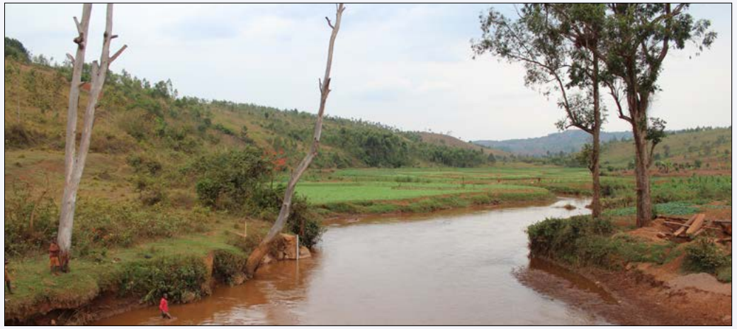
Rehabilitation and renovation of existing stations will ensure protection against vandalism and unauthorised access
