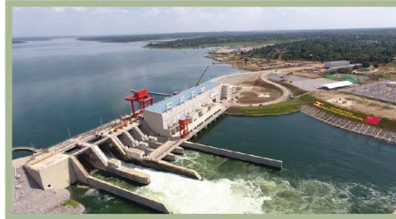
183MW Isimba Hydropower Project
