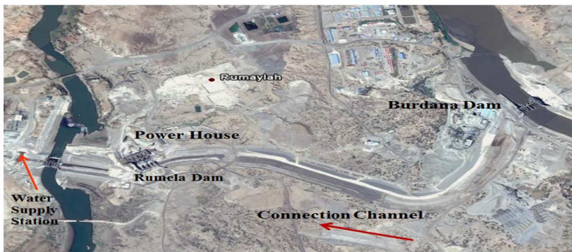
Fig (1c) Rumela, Burdana Reservoirs and the Linking Channel
