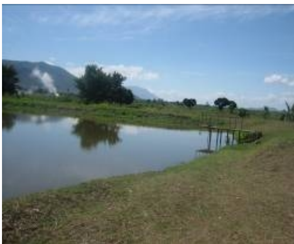
Dam for storing irrigation water
