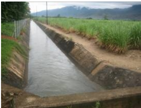
Main canal from pumping station
