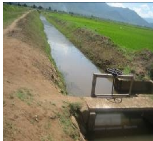
Main canal from the dam
