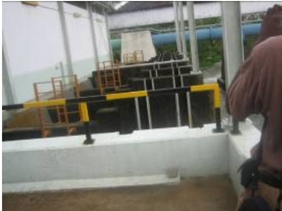
Main pumping station
