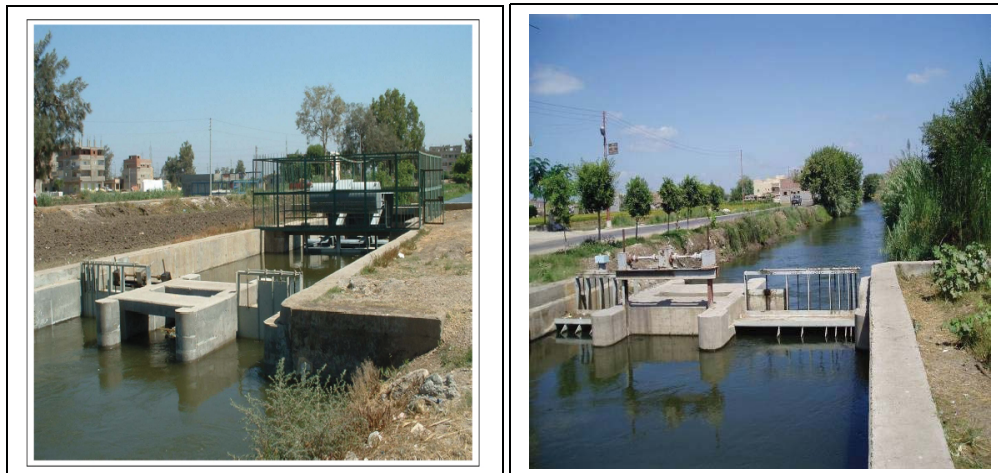
Figure 12. New Control gate in Main and Branch Irrigation Canals
