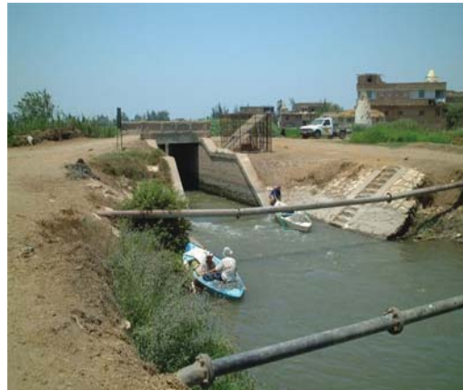
Intake of the delivery canal
