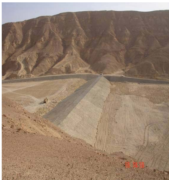
Land preparation on the site
