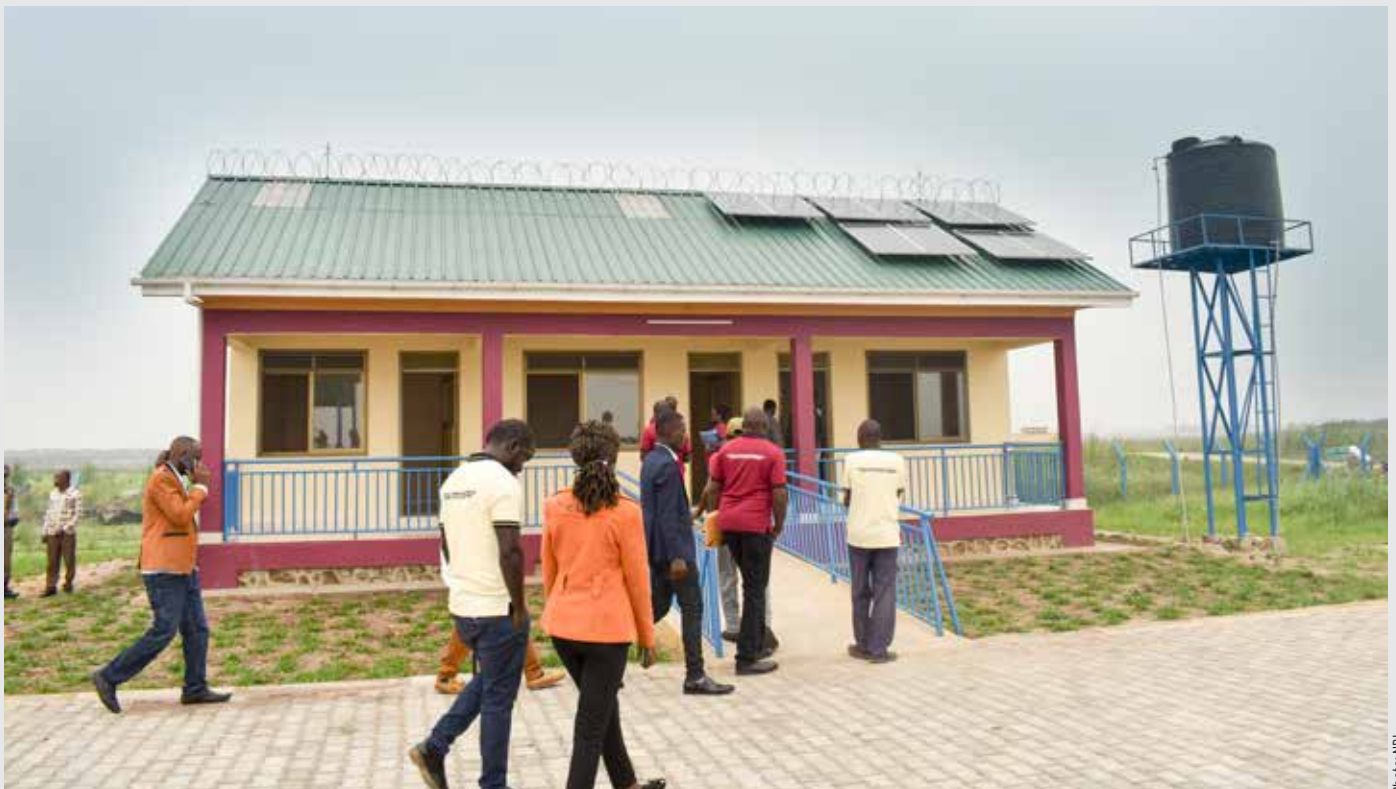
Fisheries Officers Office and Administration block at Rwenshama landing site in Uganda, constructed under LEAF II project
