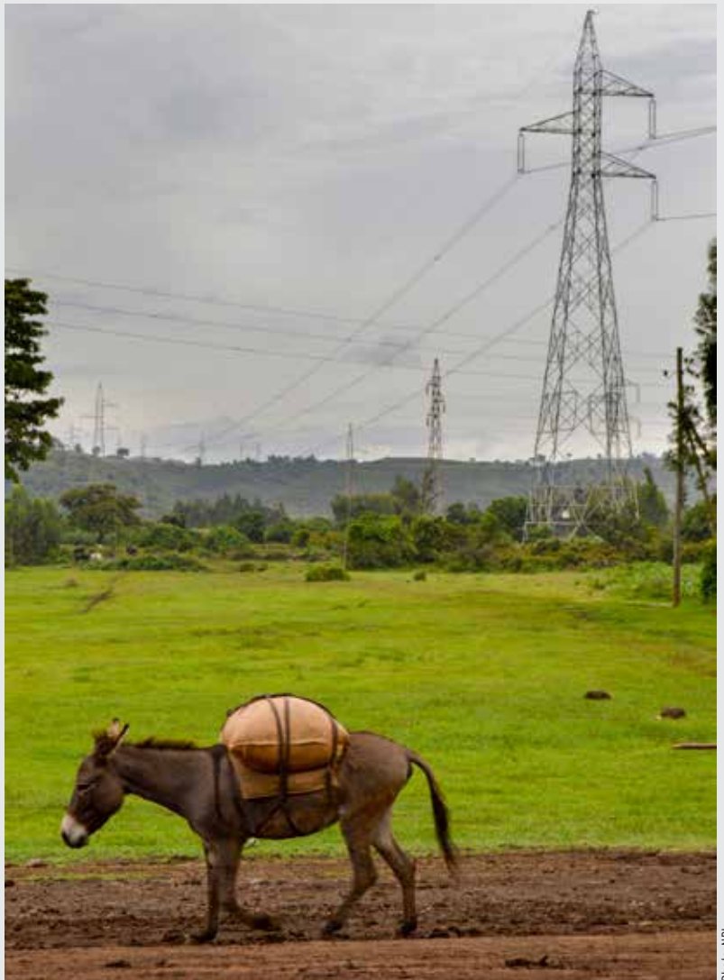
Ethiopia-Sudan Power Transmission Interconnection
