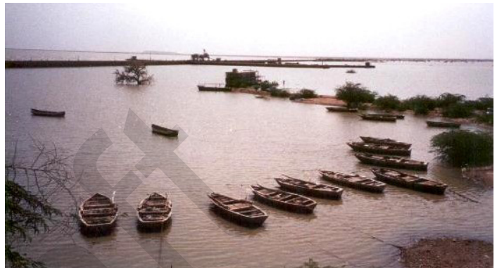
Jebel Aulia dam is located at the mouth of the White Nile. It was built in 1937 with a storage capacity of 3.5bm 3 and is used for multi-purpose ,i.e. irrigation,hydropower and flood control.
