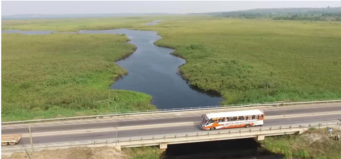
Photo 2: Bridge over the Katonga River and Katonga wetland on the Kampala-Masaka Road (Photo: Base Media)
