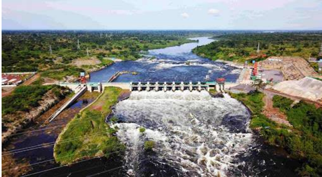
Figure 42. Karuma hydropower plant
