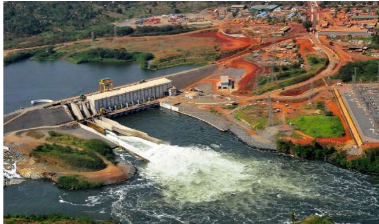
Figure 44. Bujagali hydropower plant
