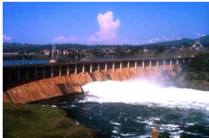
Figure 45. Owen Falls hydropower plant
