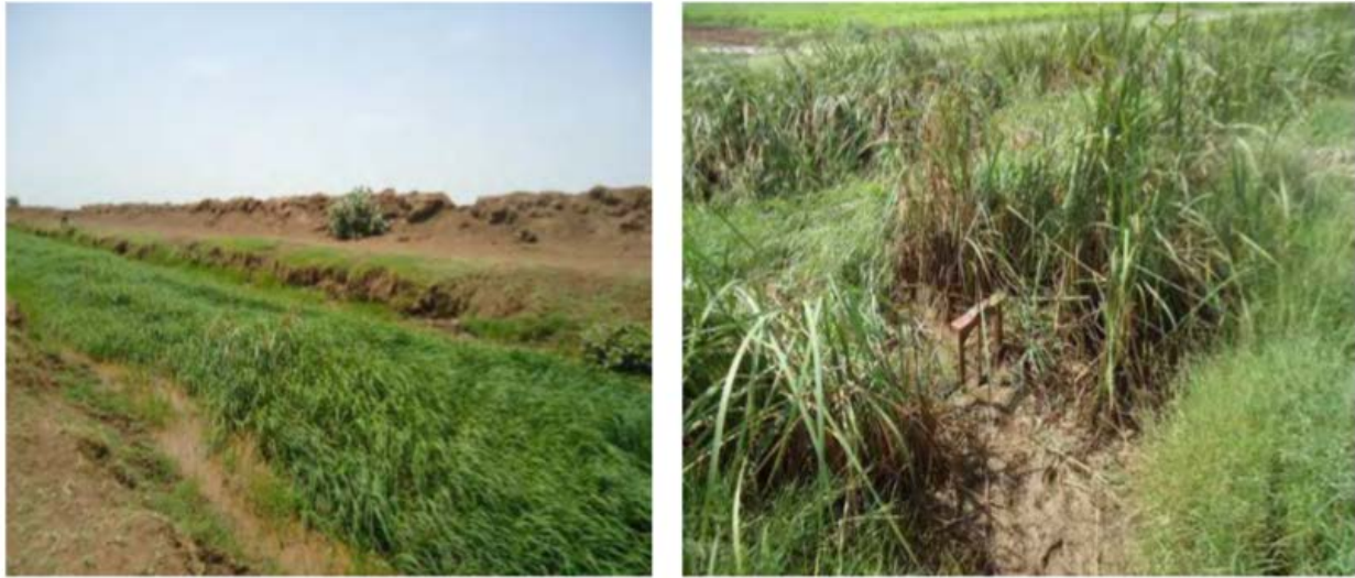
Figure 11. Weeds at the head-end and tail-ends of a minor canal (Tuweir) in the Gezira irrigation scheme in Sudan [20].
