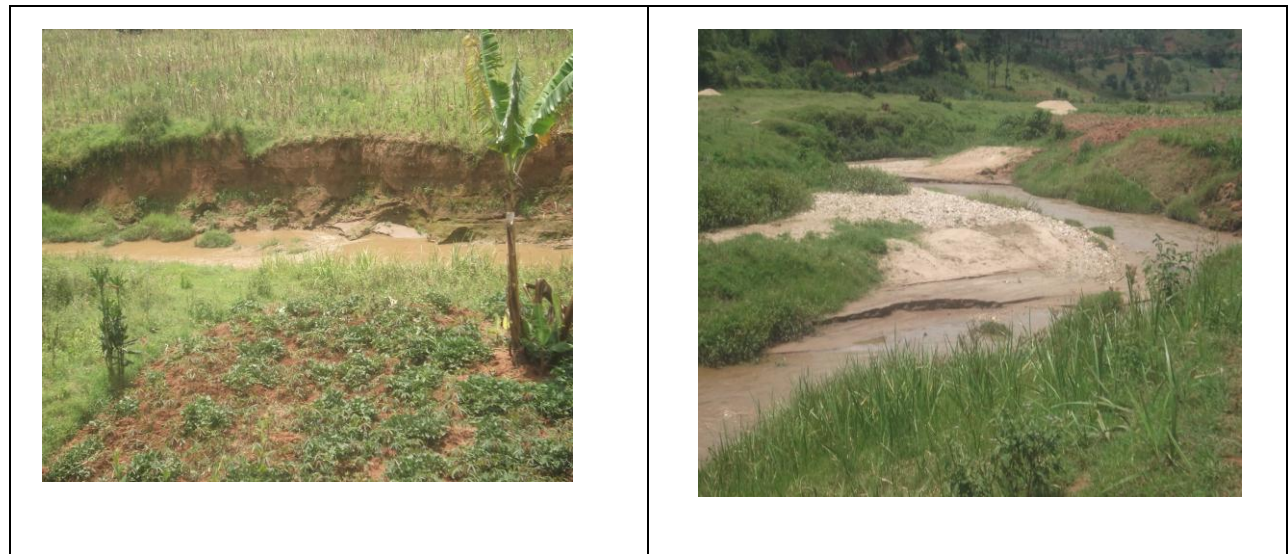
Picture 2-3: Pictures showing siltation in Mwogo River
