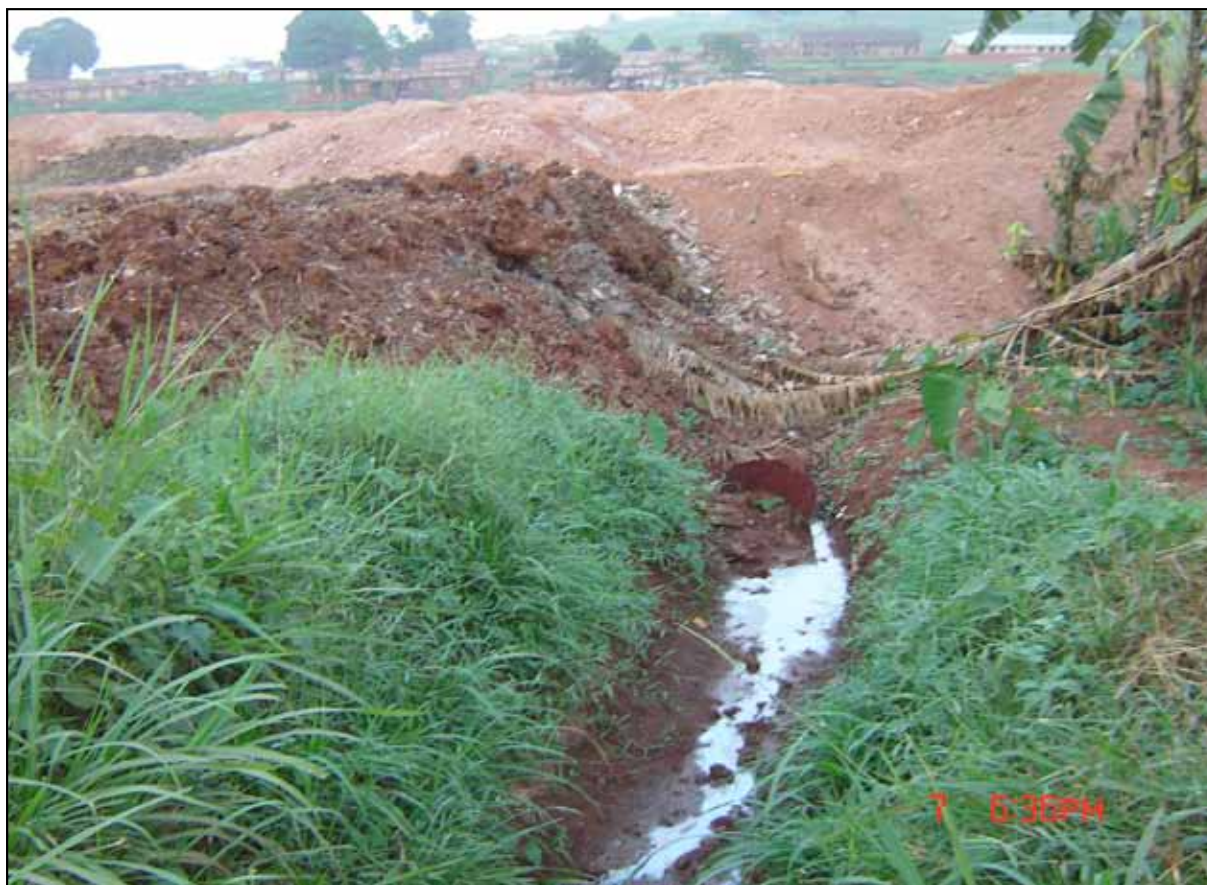
Photograph 11: Drainage channels in a wetland due to in filling can be disastrous. The channels should be made in such a way that the wetland continues to perform its functions. In this case the capacity to reduce flooding may be impaired.
