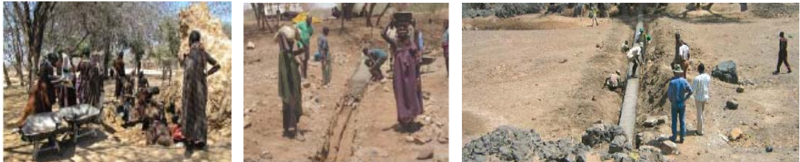
Plate 13: Subsurface dam under construction (example from Kenya)
