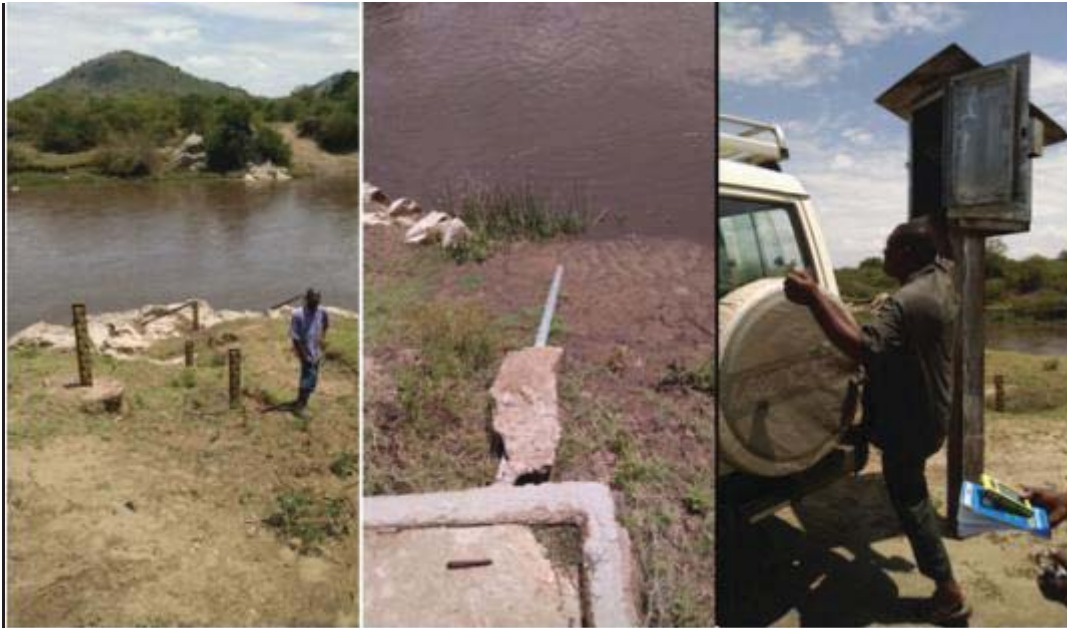
Observer standing next to staff gauges; piping protecting pressure sensor cable; housing for pressure sensor data logger
