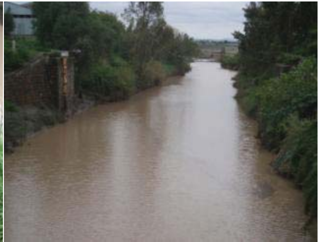
Downstream view from new bridge
