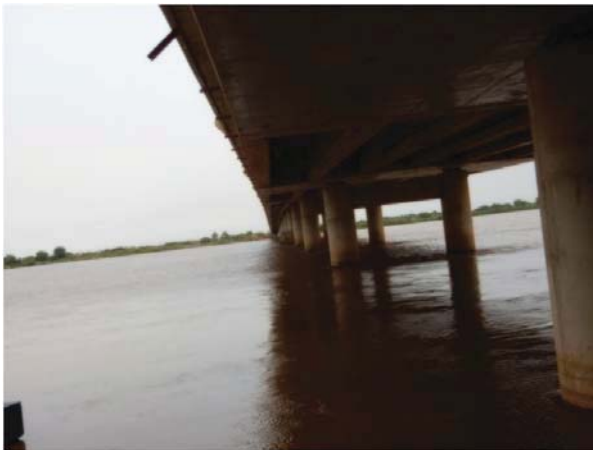
Shendi Bridge, Upstream Side
