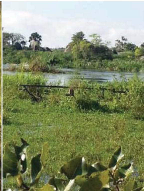
Figure 14: Remains of cable way
