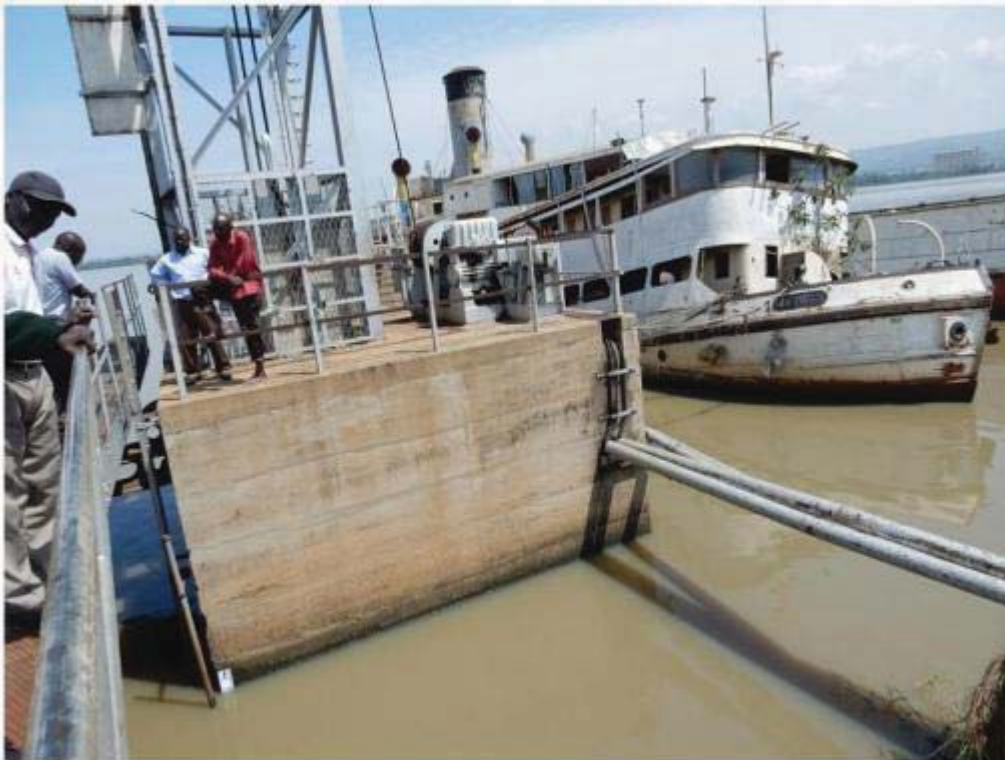
Lake Victoria Water Level Monitoring Station
