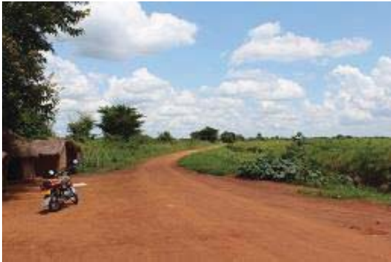
Access road to Masindi Port (pier through wetlands, blocking flow)
