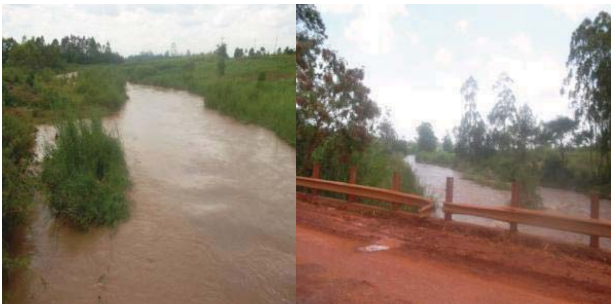
Lusumu River upstream and downstream of road bridge and Hydrometric Station
