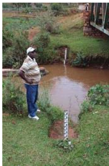
Staff gauges at Waga road bridge
