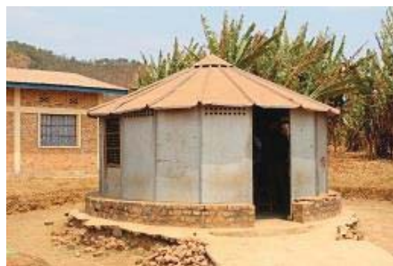
Unipod: Muriza Station Office
