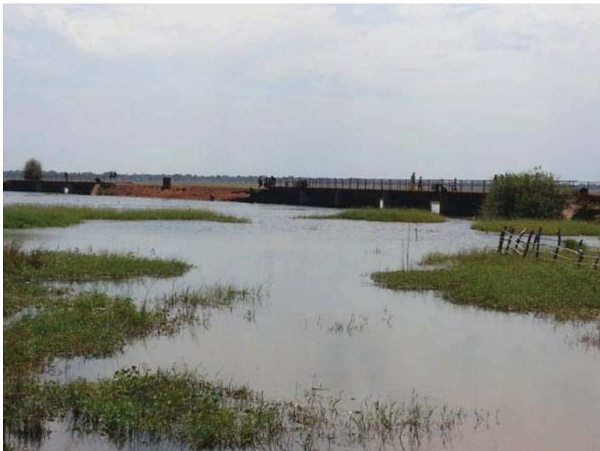
Figure 27: Partial view of downstream section below bridge
