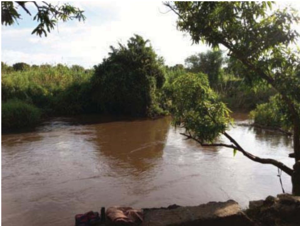
Figure 20: Pump house – intake water supply system for Torit town.
