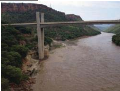
Upstream view from old bridge
