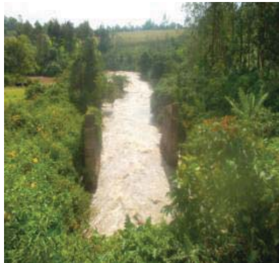
River Isiukhu downstream from bridge
