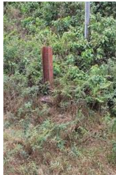
Support post of former cableway installation
