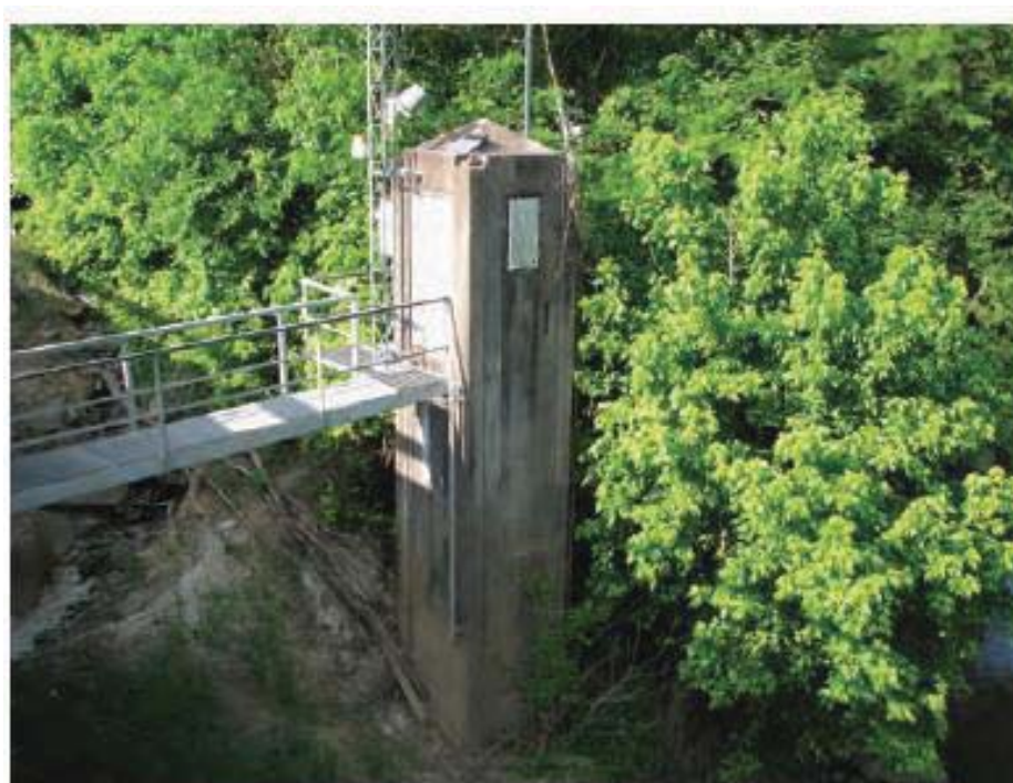
Figure 9: Recommended reinforced concrete stilling well and shelter.
