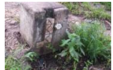
Silted up staff gauge
