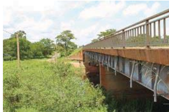
Gulu-Kampala Road Bridge at River Kafu
