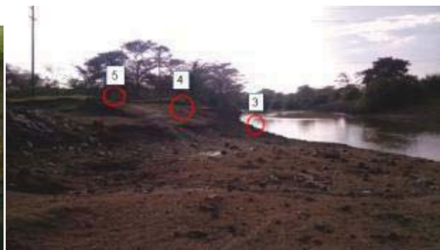
Downstream of Grumeti from bridge showing staff gauges 3-5
