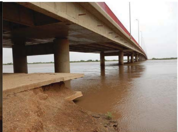
Shendi Bridge, Downstream Side
