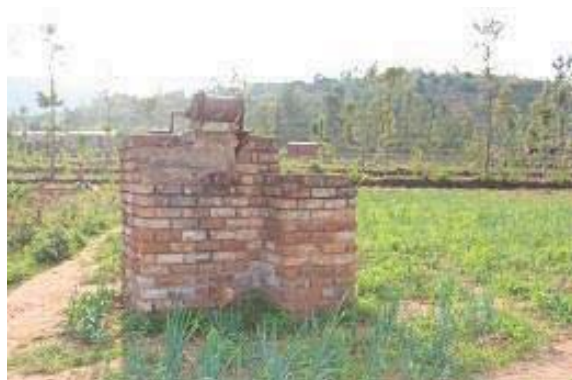
Winch for cableway system (no longer used, but in good condition)
