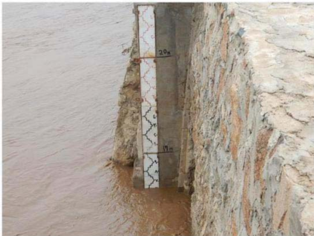
Wed Medani Manual Water Level Staff Gauge
