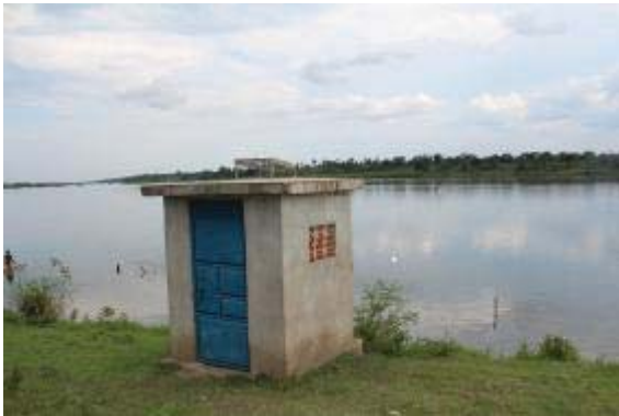
Newly constructed equipment shelter
