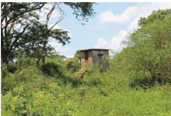
River Kafu - equipment shelter (no equipment)
