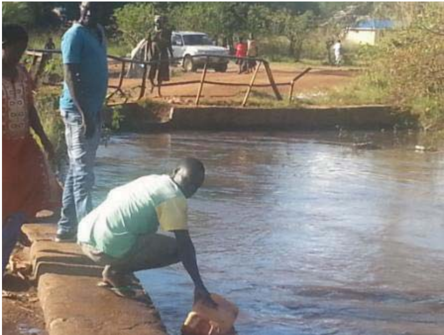
Figure 17: Bridge within Torit town.
