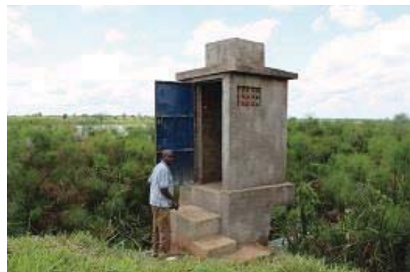
Newly constructed equipment shelter
