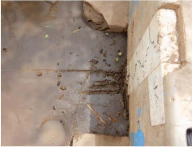
Shendi Hydrometric Station-Staff Gauge (Silt Deposit)
