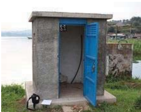
Newly constructed equipment shelter
