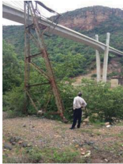
Damaged cable-way
