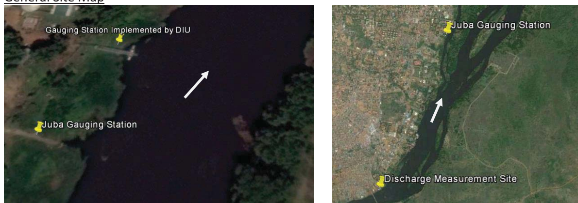
Gauging Stations at Juba Water Treatment Plant
