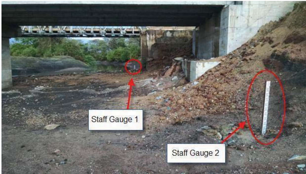
View looking upstream under new and old bridge
