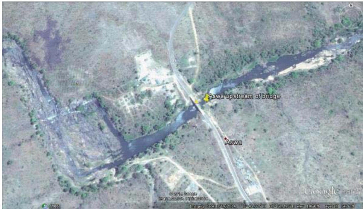
Figure 10: Aswa mouth – upstream of bridge at Juba – Nimule road.
