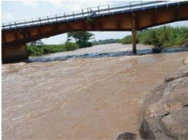
Nzoia River Bridge downstream of Station
