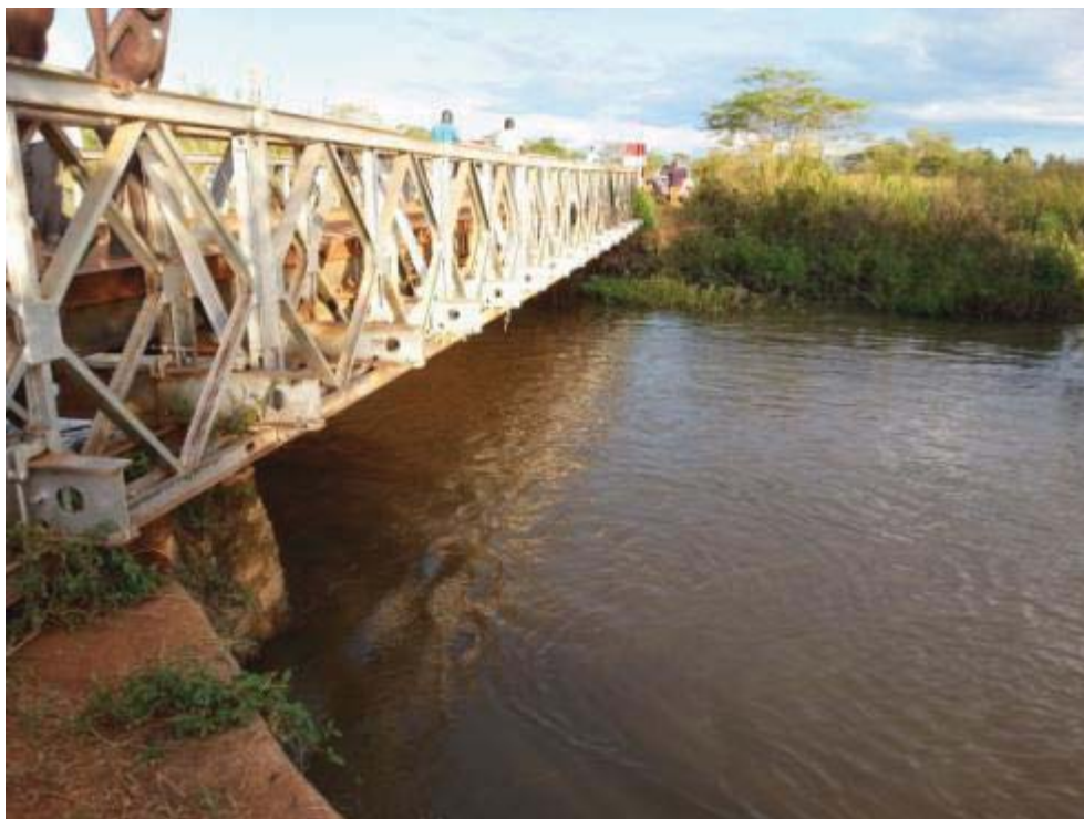
Figure 16: Upstream section of bridge; Juba-Torit road.
