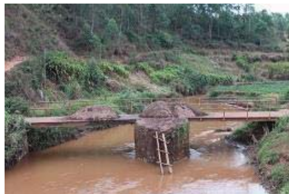
Sand mining at old bridge: no stable rating curve
