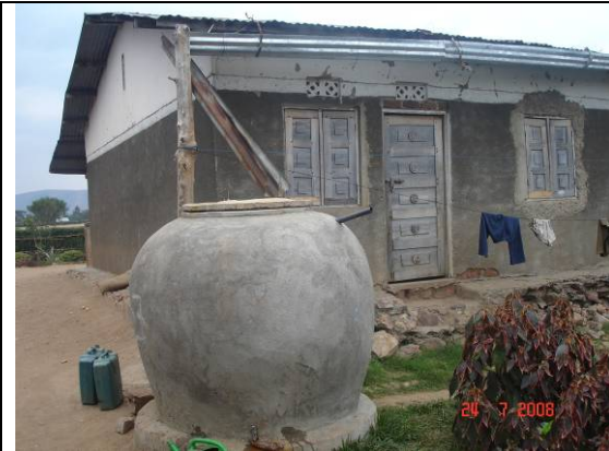
RHEPI through microgrants demonstrates rain water harvesting at Kagitumba (cross-border project with Uganda)
