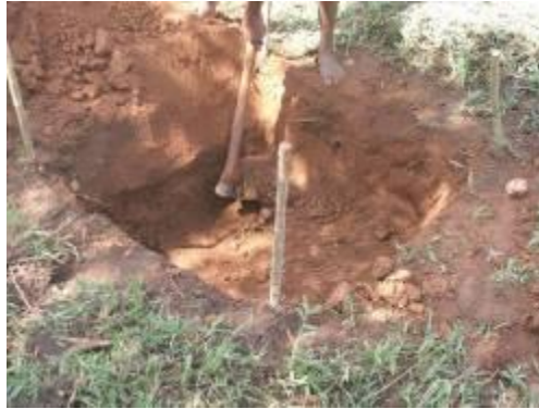
Picture 4-28: Photo of test pit
