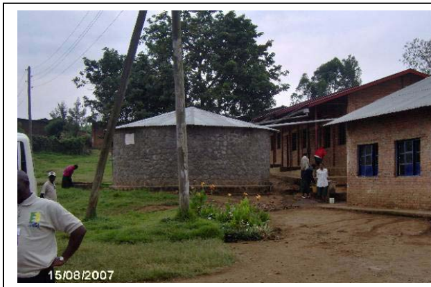
Rain water catchment tank
