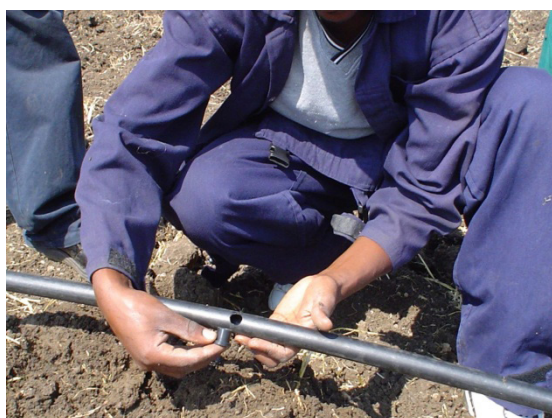
Figure 6.7 (a) Fixing emitters onto a drip lateral (photo by G. Alemu)
