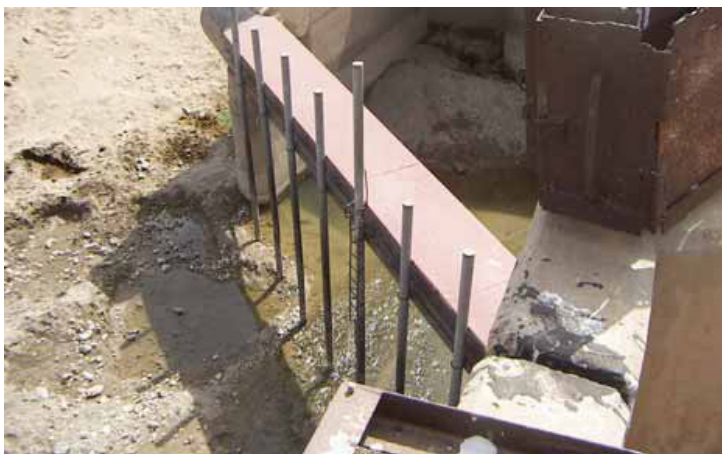
Figure 8.4 Trash deflector at canal intake ( source: FAO, 2010 )
