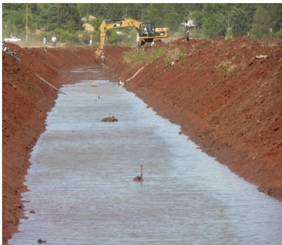
Figure 4.1 (a) Canal de-silting improves its efficiency (Photos by B. Mati)
