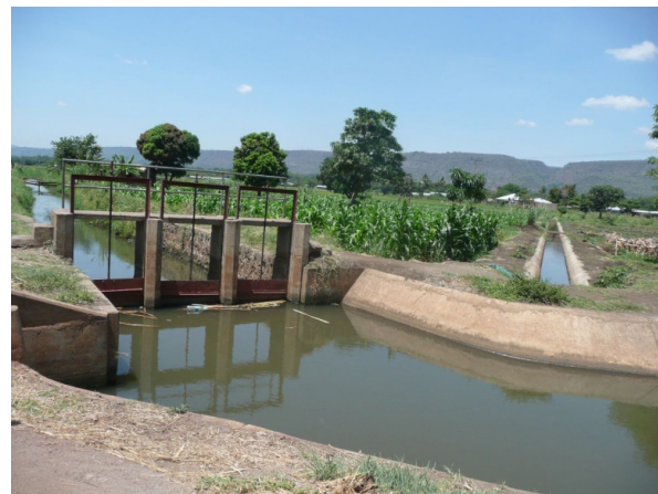
(b) Concrete lined canal reduces seepage losses
