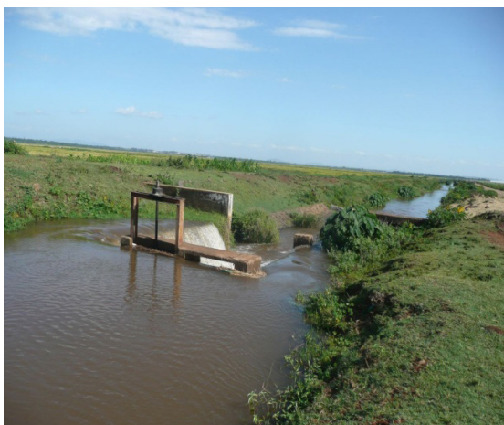
Figure 4(a) Water delivery using canals has higher losses (Photos by B. Mati)
