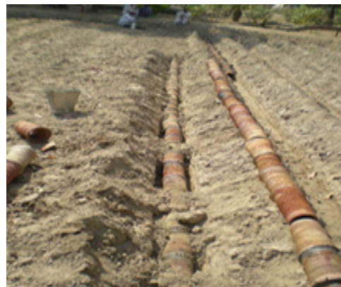
(b) Installation of clay pipes in trenches
