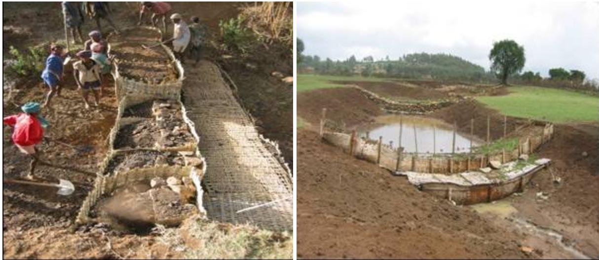
Plate 6. Check-dams constructed out of organic boxes (bamboo and reed mat)
