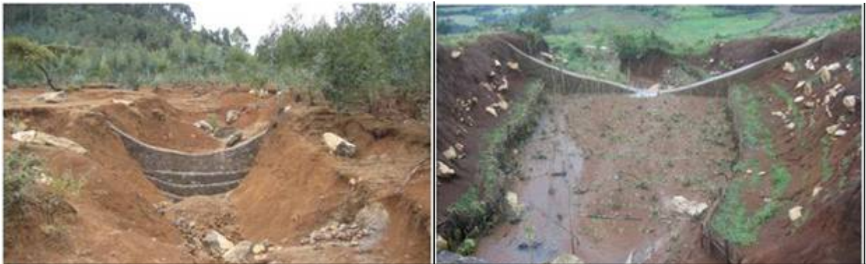
Plate 5. Well constructed arc-weir and its effect on sediment trapping
