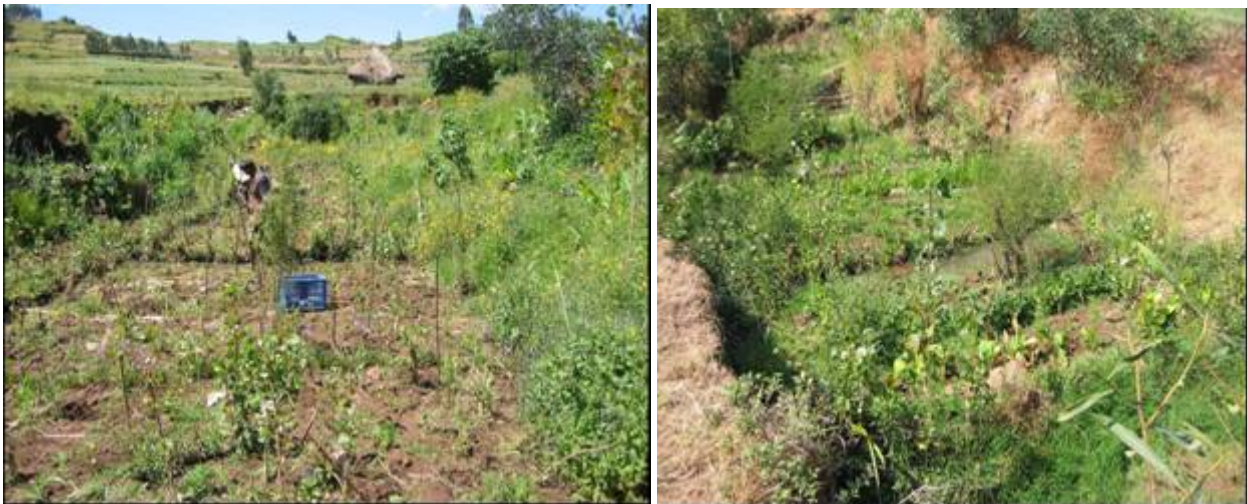
Plate 12. Gully bed and sidewall planted with various tree, bush/shrub and grass species
