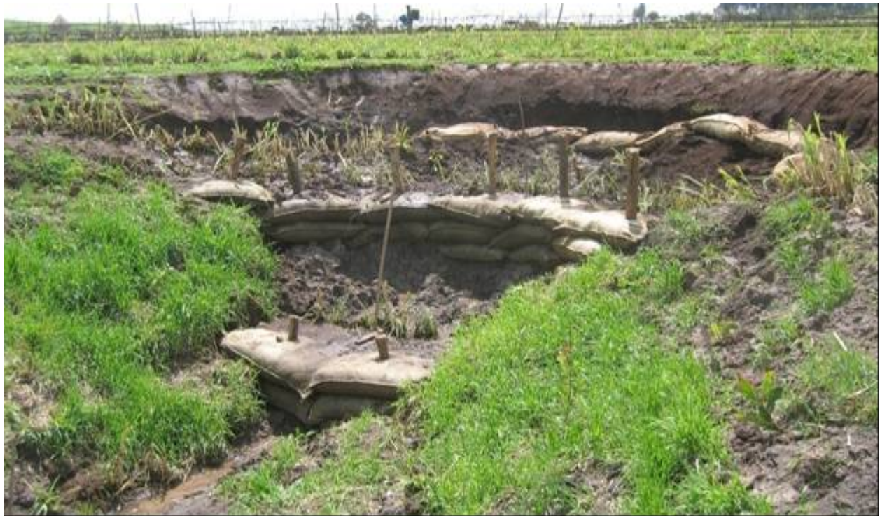
Plate 3: Gully head control with sand bags and other vegetative measures.
