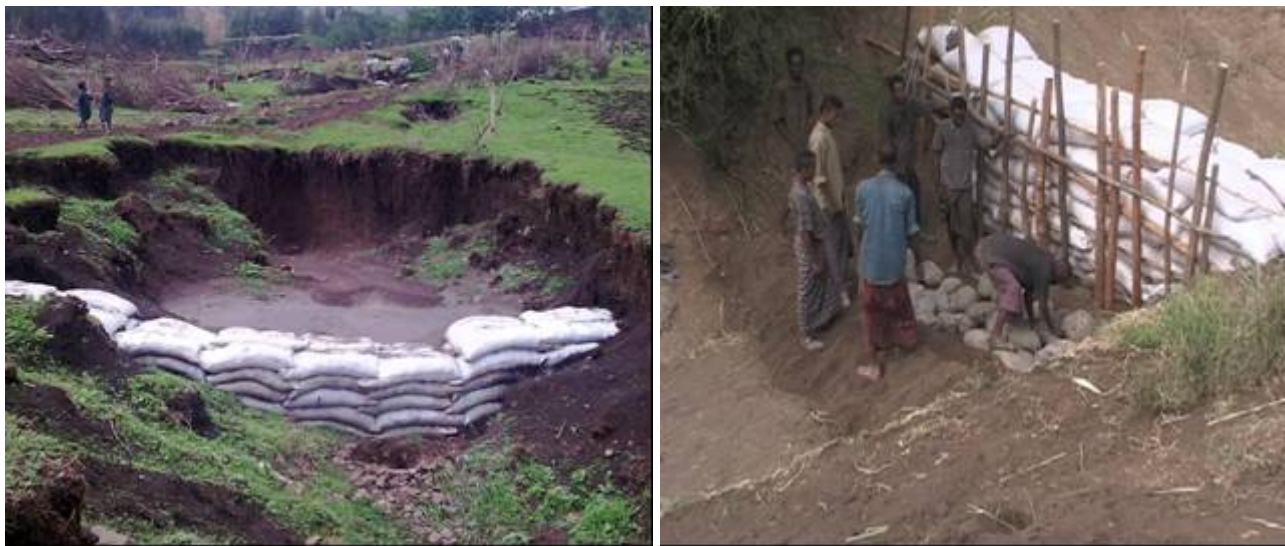
Plate 8. Sandbag check-dams constructed to treat medium sized gullies
