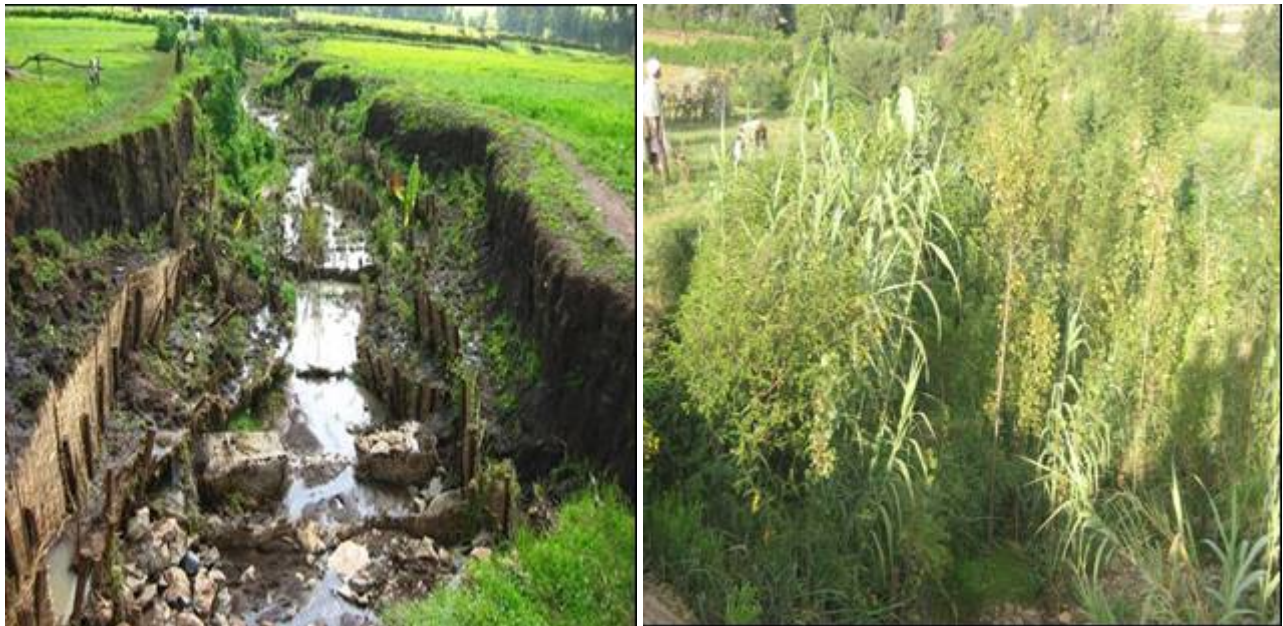
Plate 13. Protecting gully sidewall using bamboo-mat retaining wall.
