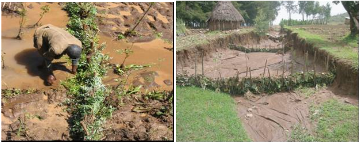
Plate 10. Bundles put across the gully bed and supported with poplar and willow stems
