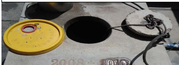
Water cellar for storing rainwater
