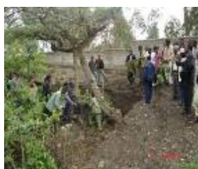
Plate (7): Brushwood Construction
