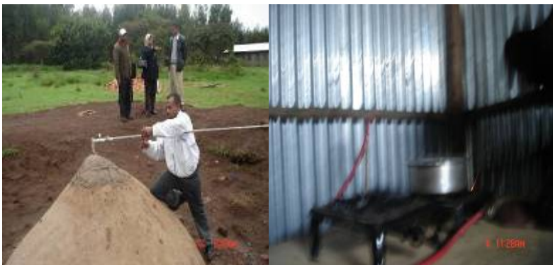
Plate (6): Biogas Construction
