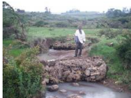
Plate (4): Gully Erosion Control
