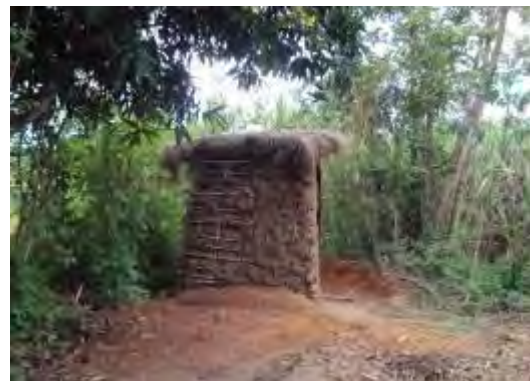
Figure 6-46: Typical latrine in the project area
