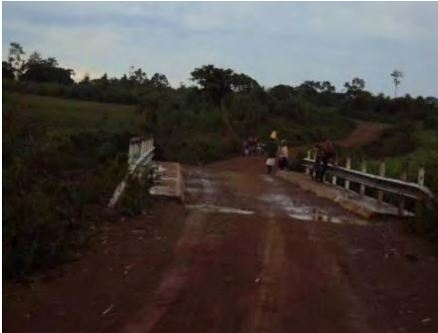
Figure 6-48: Lugulu –Namisi Road and Bridge in the project area
