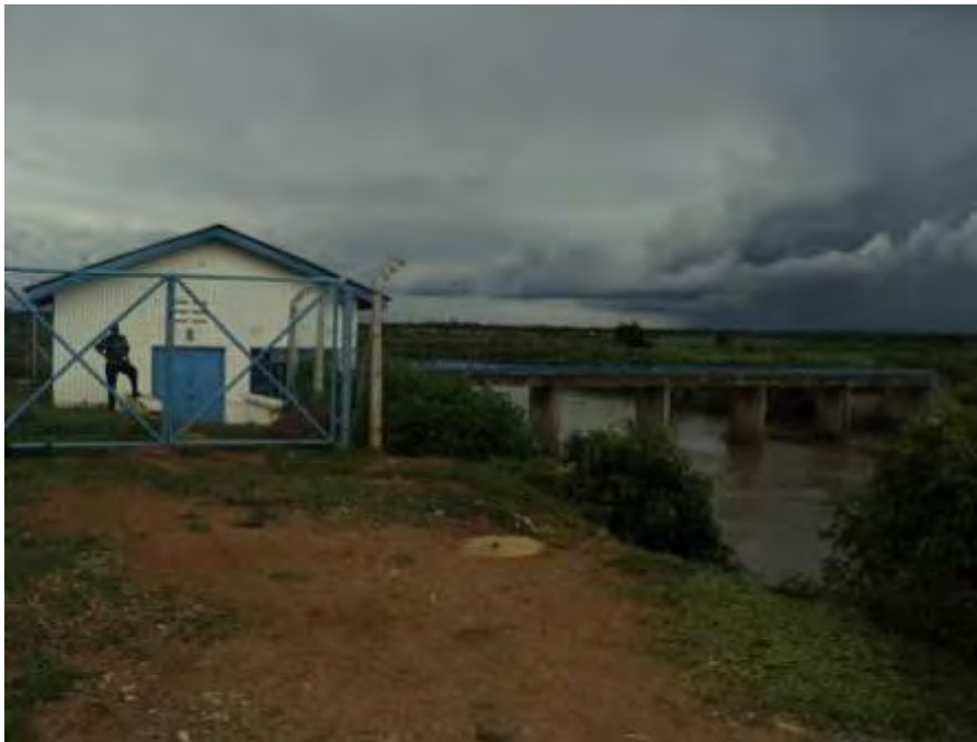
Figure 6-18: Abstraction point for Busia-Mundika Water Supply system on River Sio
