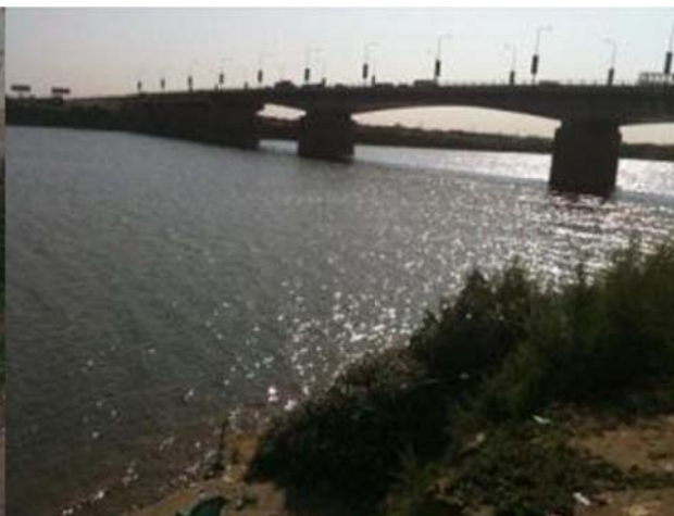
Figure 3. Manshiya bridge monitoring station
