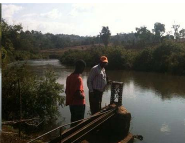
Figure 5. Sor damaged cableway
