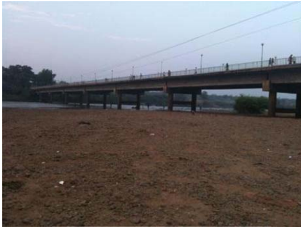
Figure 8. Baro bridge at Gambella
