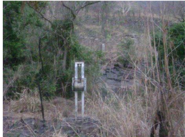
Figure 7. Installation for cableway
