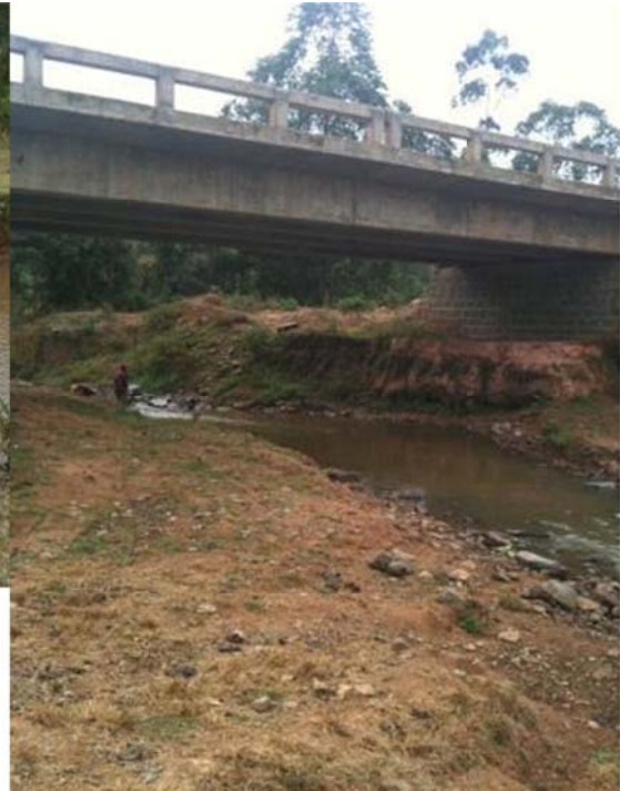
Figure 13. Bridge over Oka
