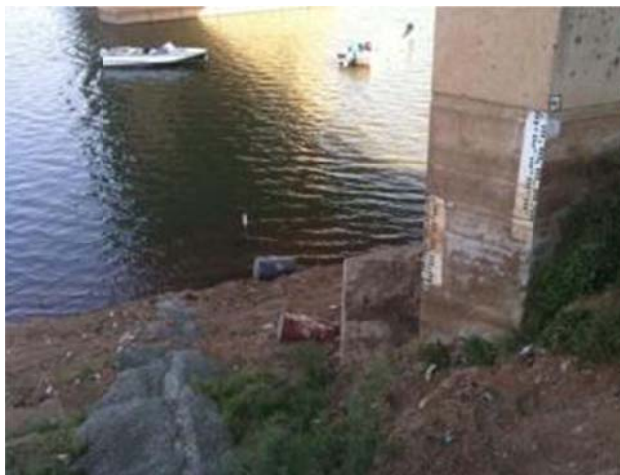
Figure 2. Magnimir monitoring station
