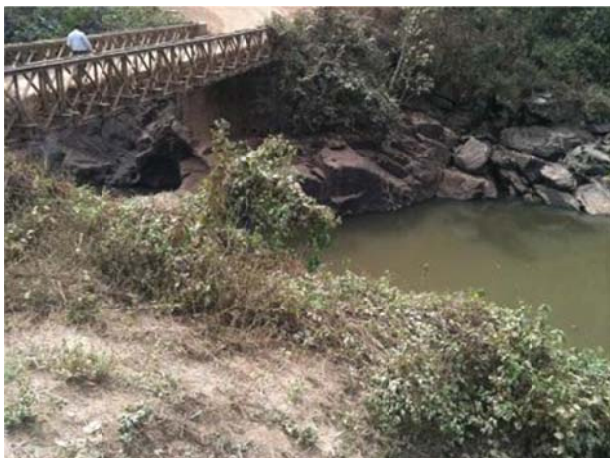
Figure 14. Bridge over Geba
