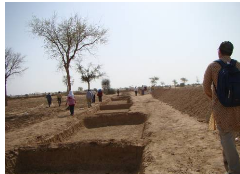
Field trenches and bunds to harvest rainwater
