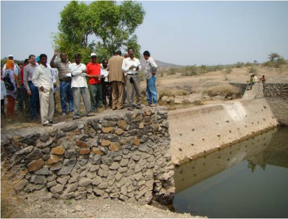
The masonry check dam, Boltek watershed
