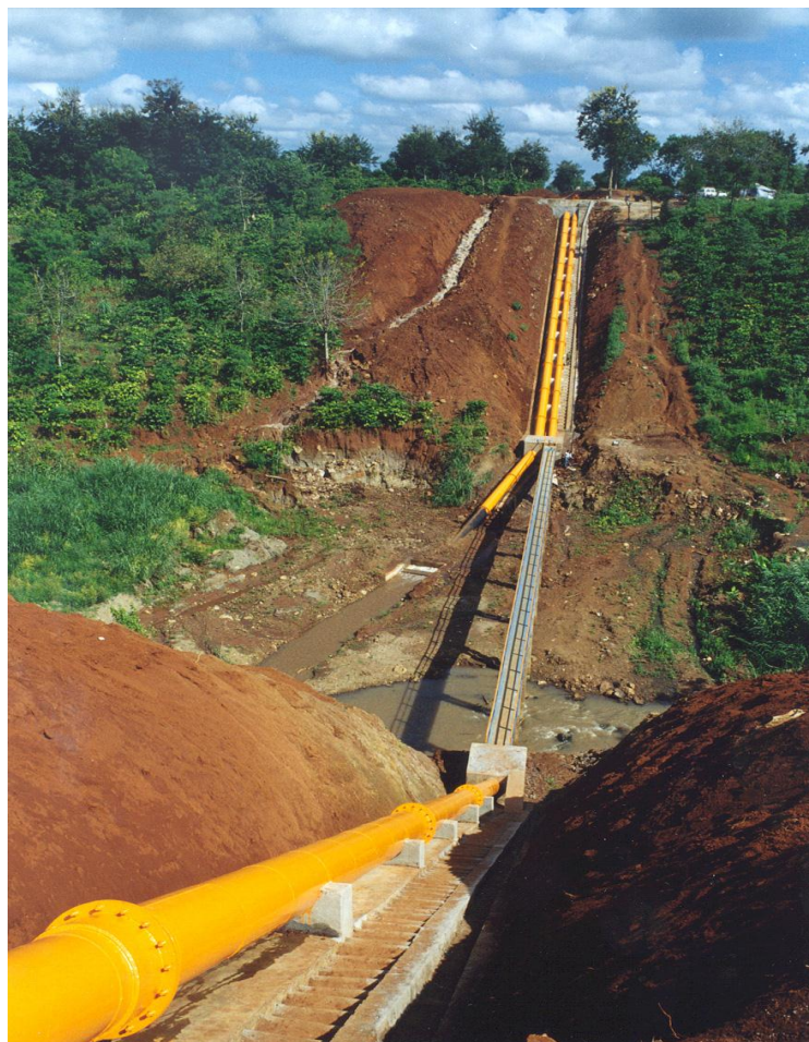
Photograph 1.3: Inverted Siphon Crossing of River Channel (Dak Lak, Vietnam)
