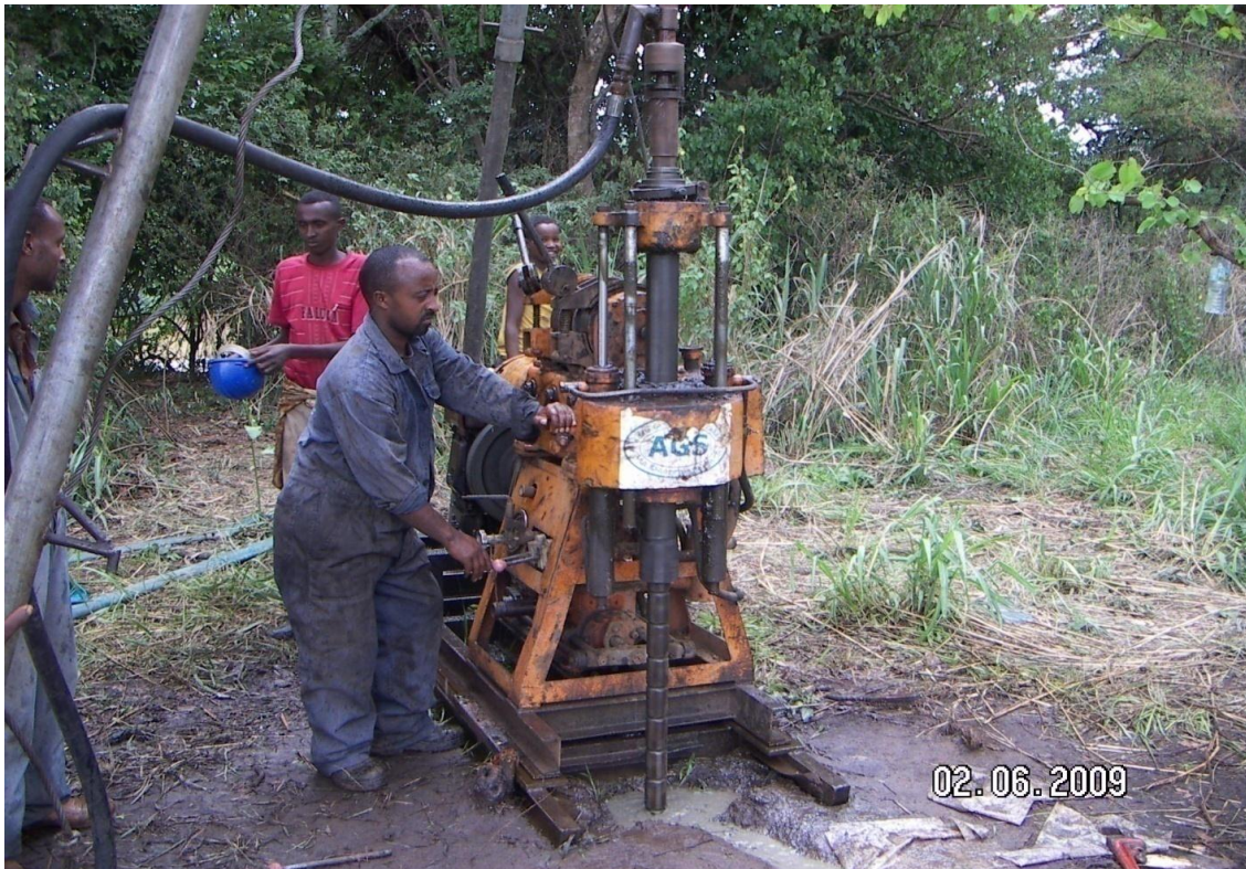
Plate 6.2: Drilling on progress at Borehole no DWBH - 1
