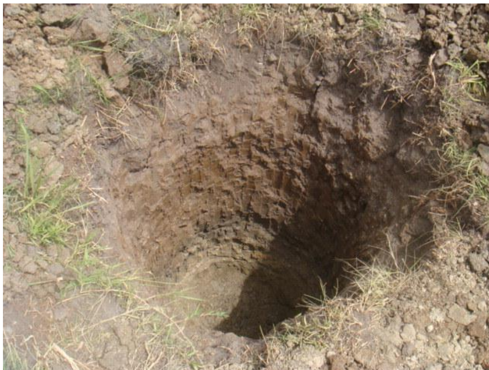
Test pit in feeder canal alignment
