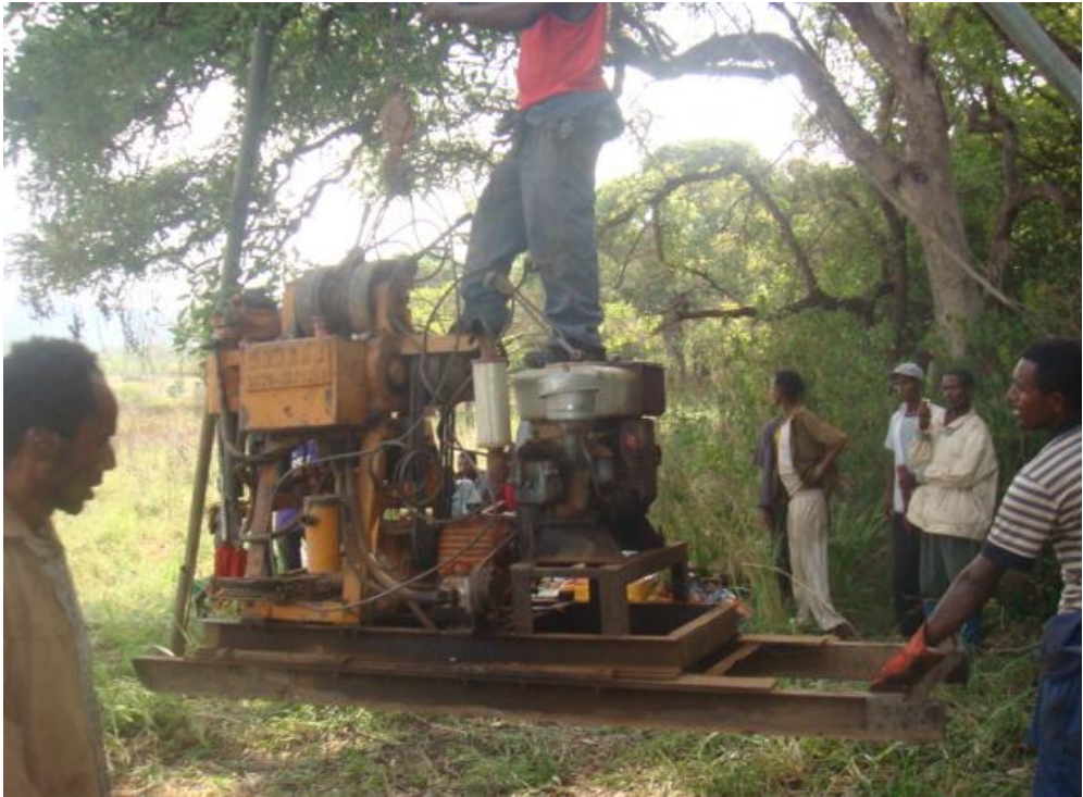
Skid mounted rig
