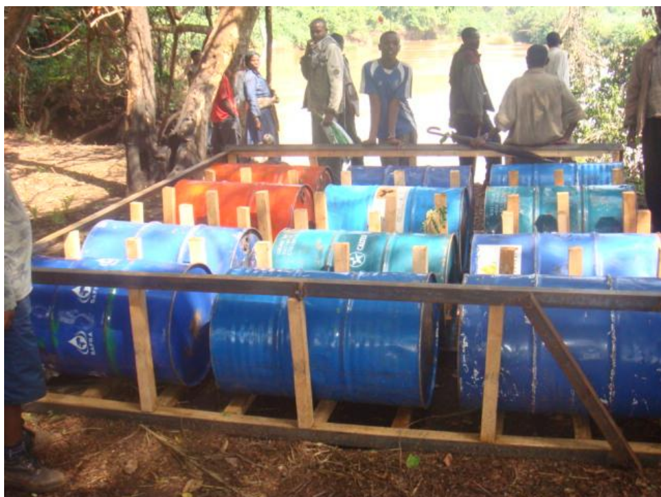
Assembling raft on left bank at diversion site
