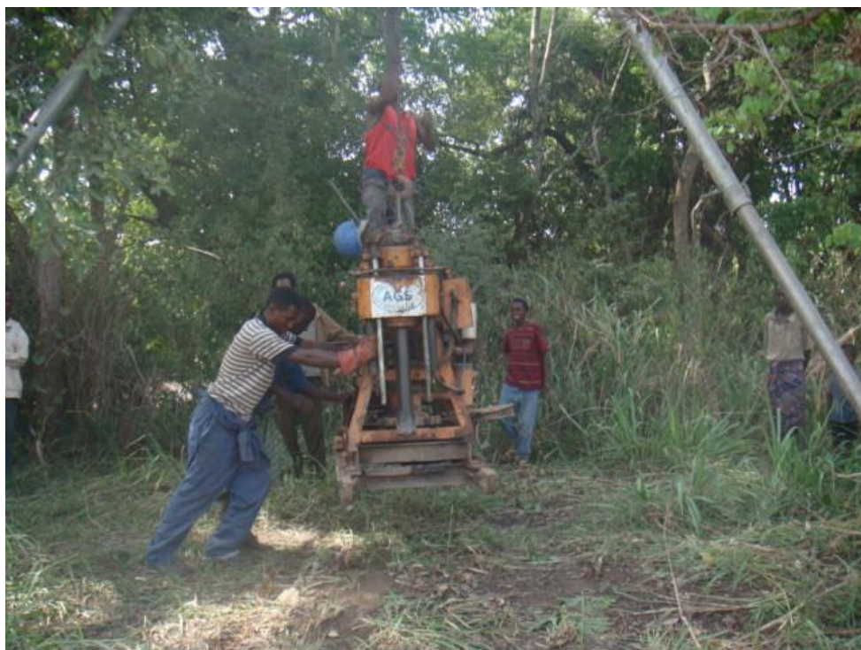
Off loading rig
