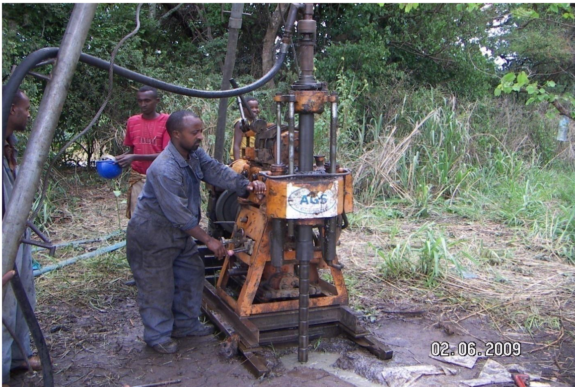
Figure 1. Core drilling operation at DWBH-1 (left bank)
