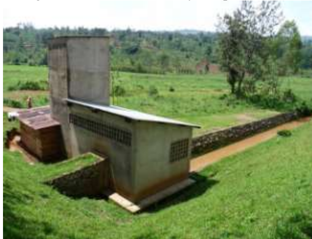
Figure 33: micro Kiremba hydro- power house
