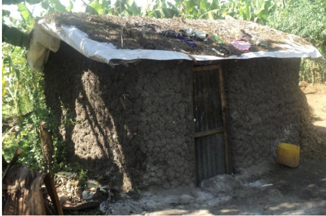
Figure 5-2: Residential Structure in the Proposed area for the Reservoir
