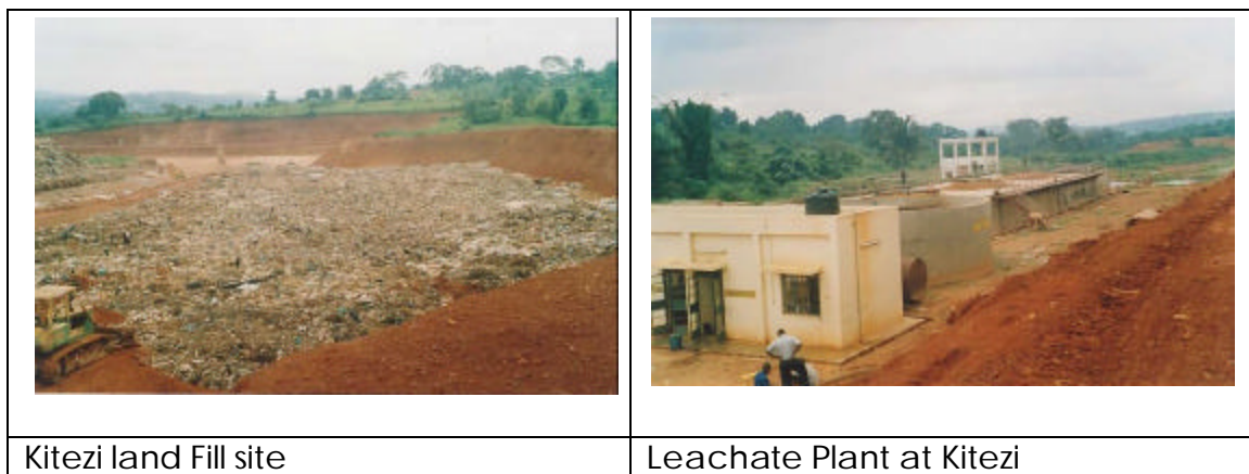
Figure 4.5: KCC waste landfill and leachate treatment plant at Kitezi (Photo by Moses Otim, January 2005)
