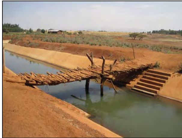
Photo 5-2: Informal bridge over new canal in Koga Irrigation Project
