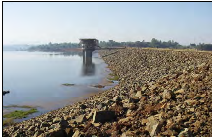
Photo 4-32: Koga Dam and reservoir
