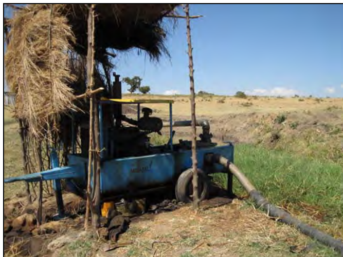
Photo 4-15: Commercial irrigation by pump from Dirma River: Wawa Farm, 2009
