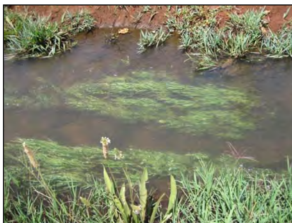
Photo 5-3: Weed growth in new channel in Koga Project
