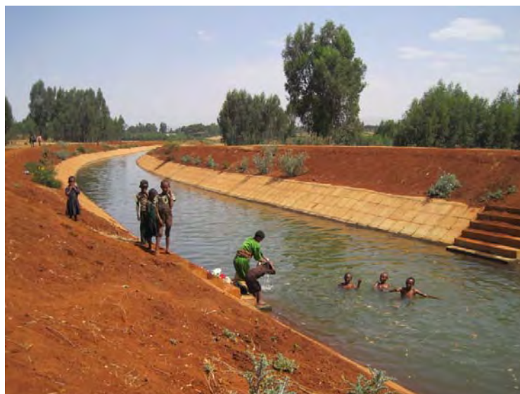
Photo 5-6: Washing and swimming in new canal in Koga Irrigation Project
