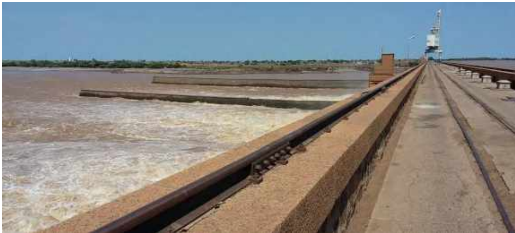
Figure 23: Sennar Dam at Blue Nile, view downstream
