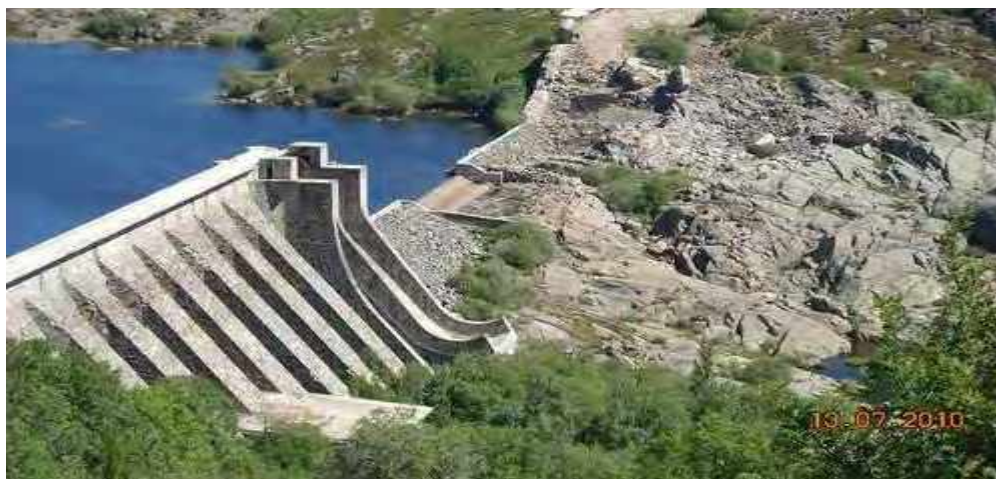
Figure 34: Vega de Tera Dam after failure
