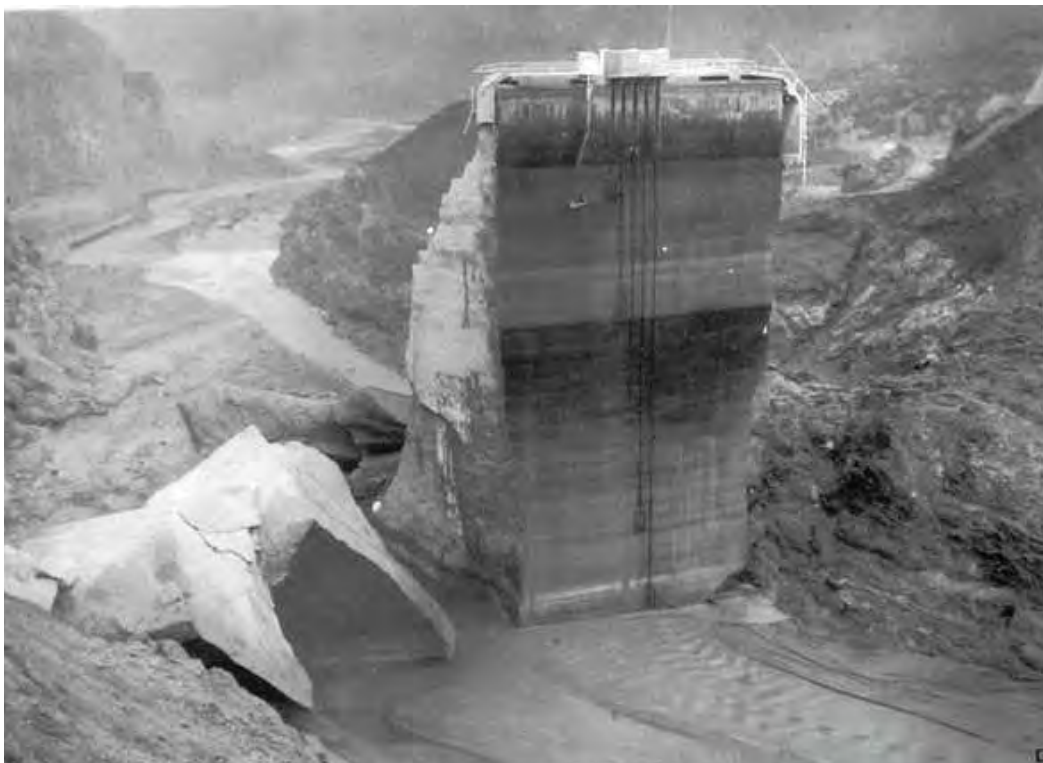
Figure 28: St Francis Dam after failure
