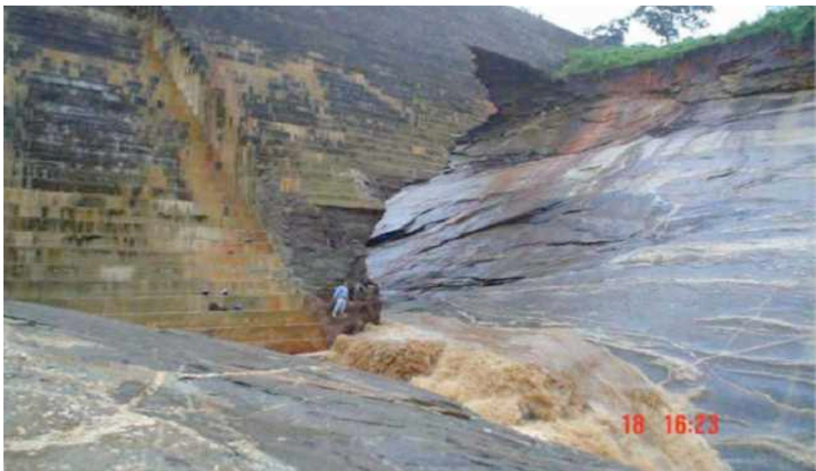
Figure 26: Camara Dam after failure
