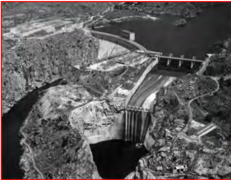
Figure 23: Aerial view of Ricobayo Dam
