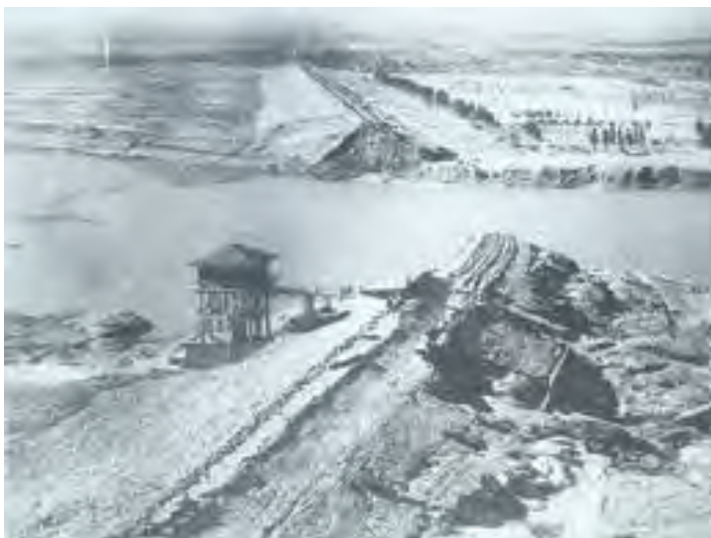
Figure 22: Banqiao Reservoir Dam after overtopping failure
