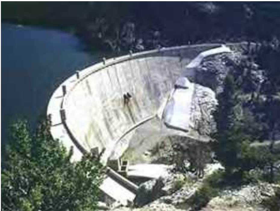
Figure 21: Gibson Dam after some remedial work
