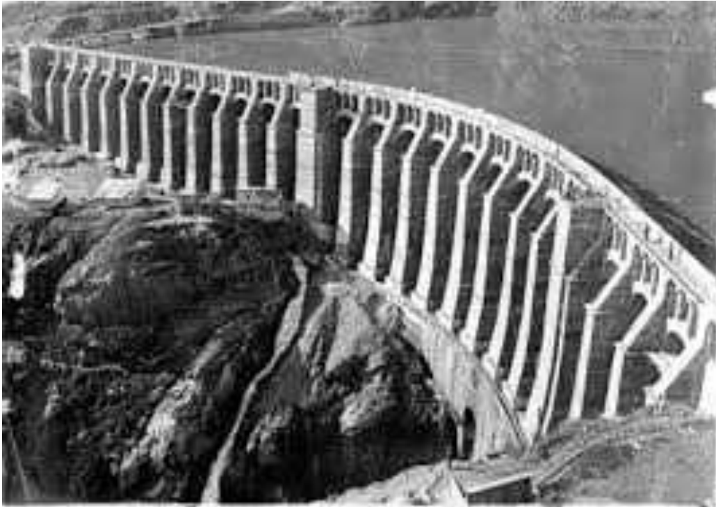
Figure 32: Gleno Dam before failure
