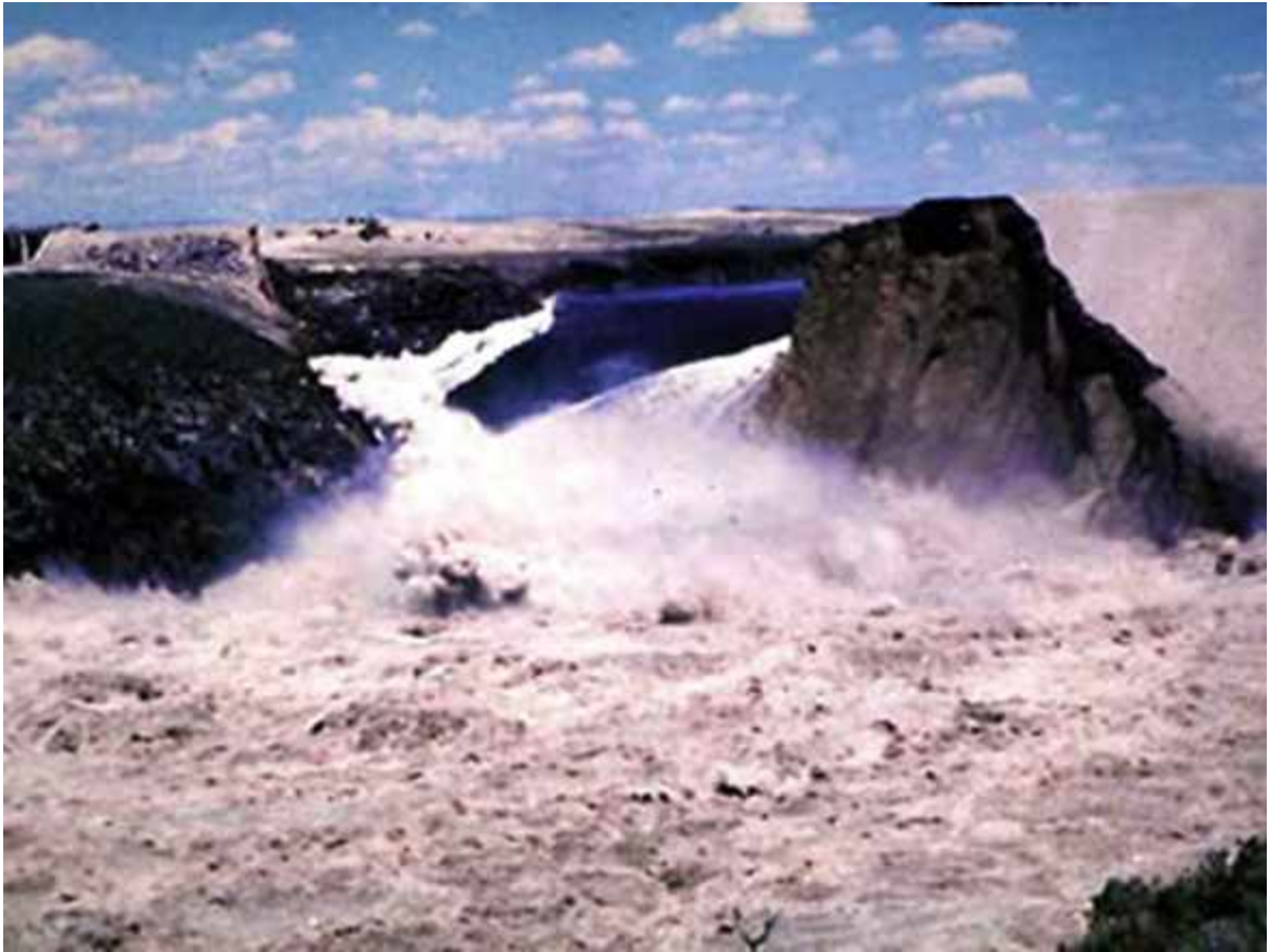
Figure 6: Teton Dam during failure
