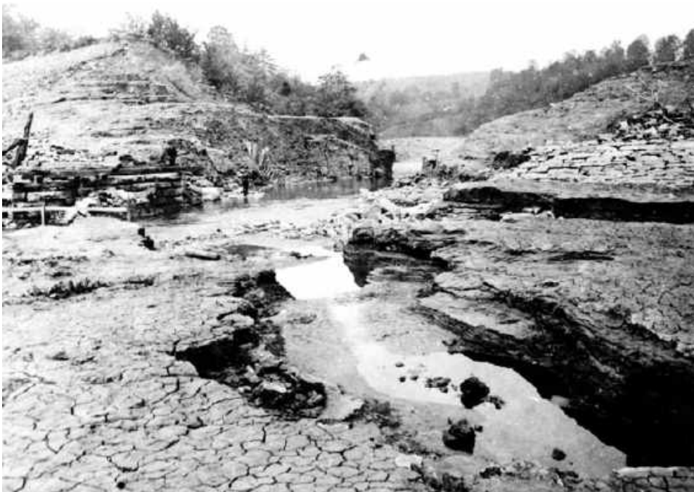
Figure 19: South Fork Dam after overtopping failure
