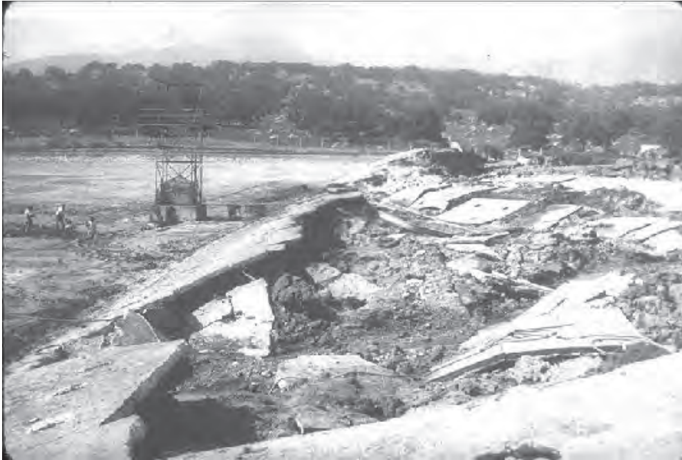
Figure 11: Sheffield Dam after seismic failure
