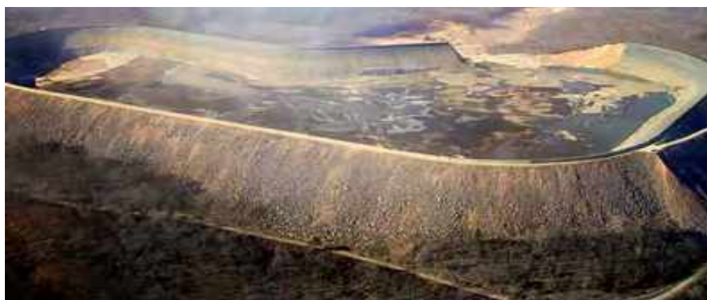
Figure 38: Taum Sauk Dam after failure
