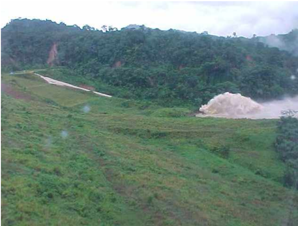
Figure 13: Sweepout of spillway stilling basin
