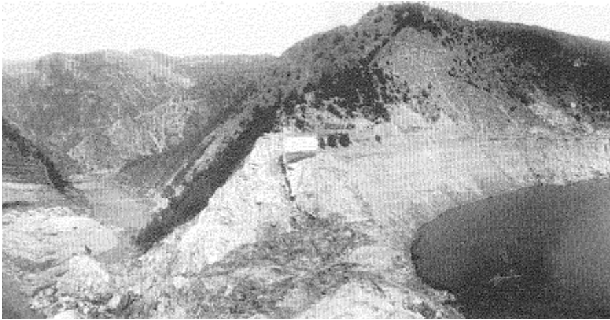
Figure 20: Secondary Dam of Sella Zerbino after overtopping failure
