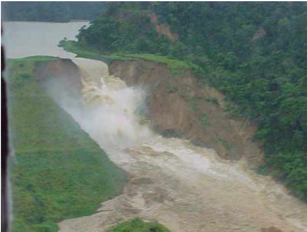
Figure 17: Breach Formation Nearing Completion
