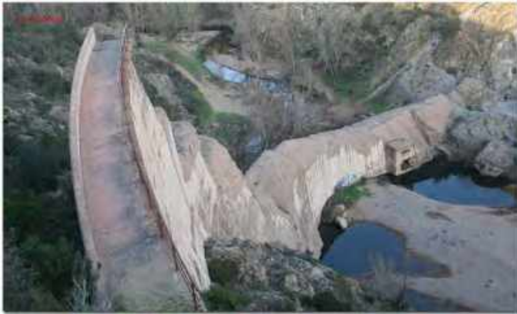
Figure 30: Malpasset Dam as it looks nowadays
