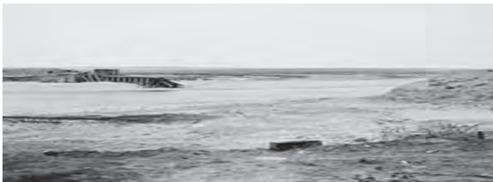
Figure 7: Avalaon Dam after its 1904 internal erosion failure
