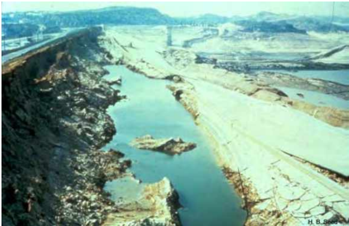
Figure 10: Lower San Fernando Dam after failure
