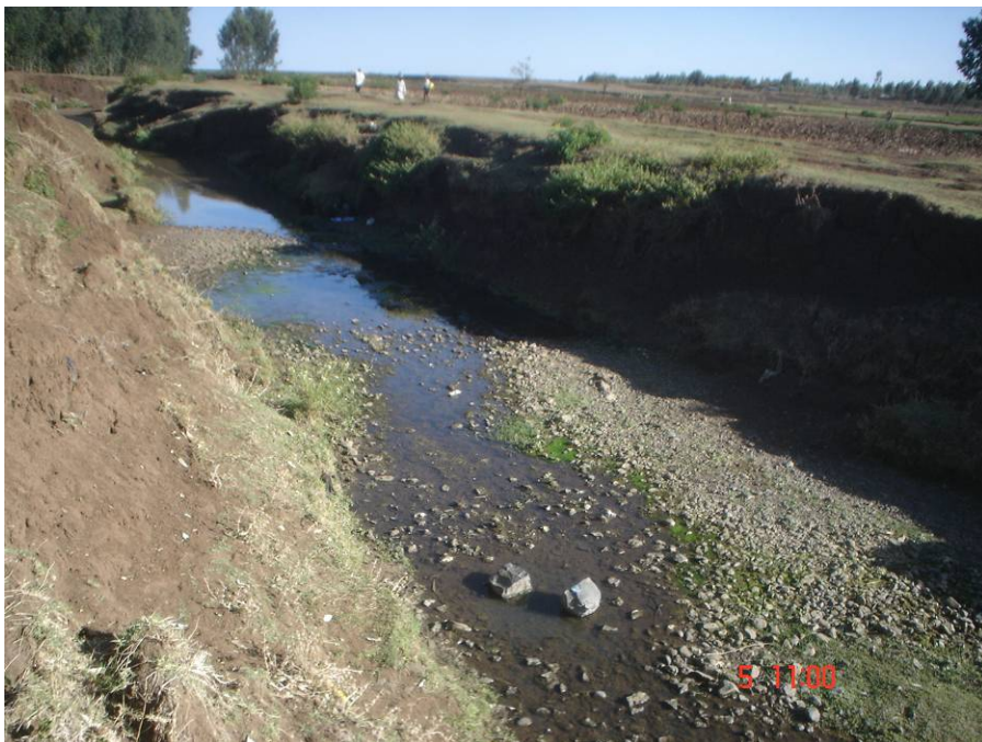
Figure 6-16: Photo of downstream Dirma River.
