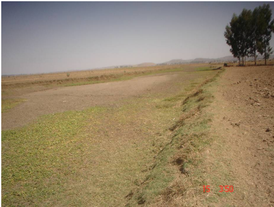
Figure 6-20: Photo of the downstream section of Ribb, showing clean channel with less vegetation.
