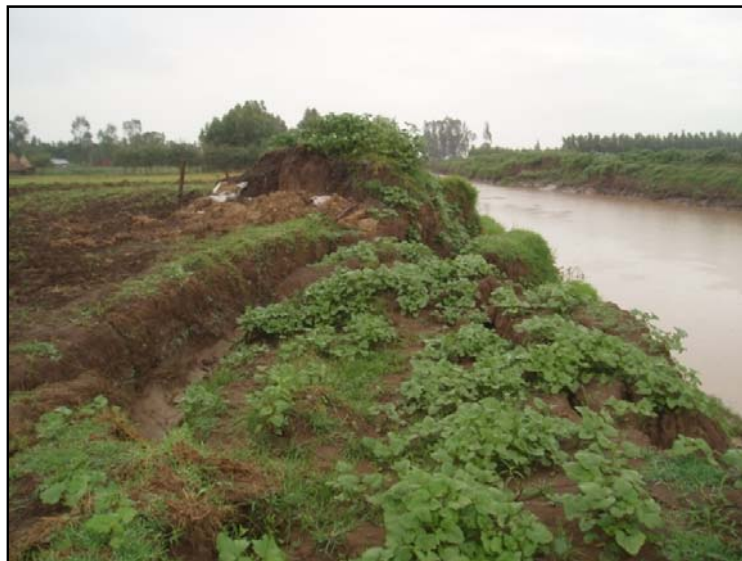
Figure 4-17: Sliding Failure of River Bank at Ribb River at the Bridge Site, (Source: Consultant Field Visit, 2009)
