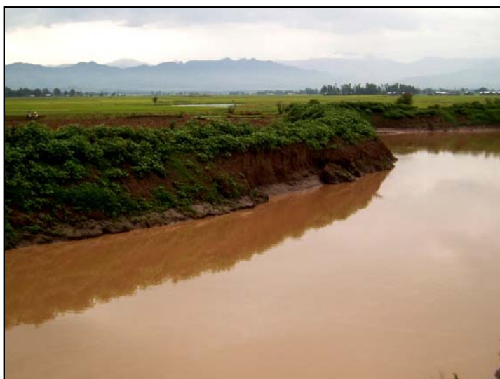
Figure 2-2: River Bank Erosion on Ribb River @ Upstream of the Main Bridge (Source: Consultant Field Visit 2009)
