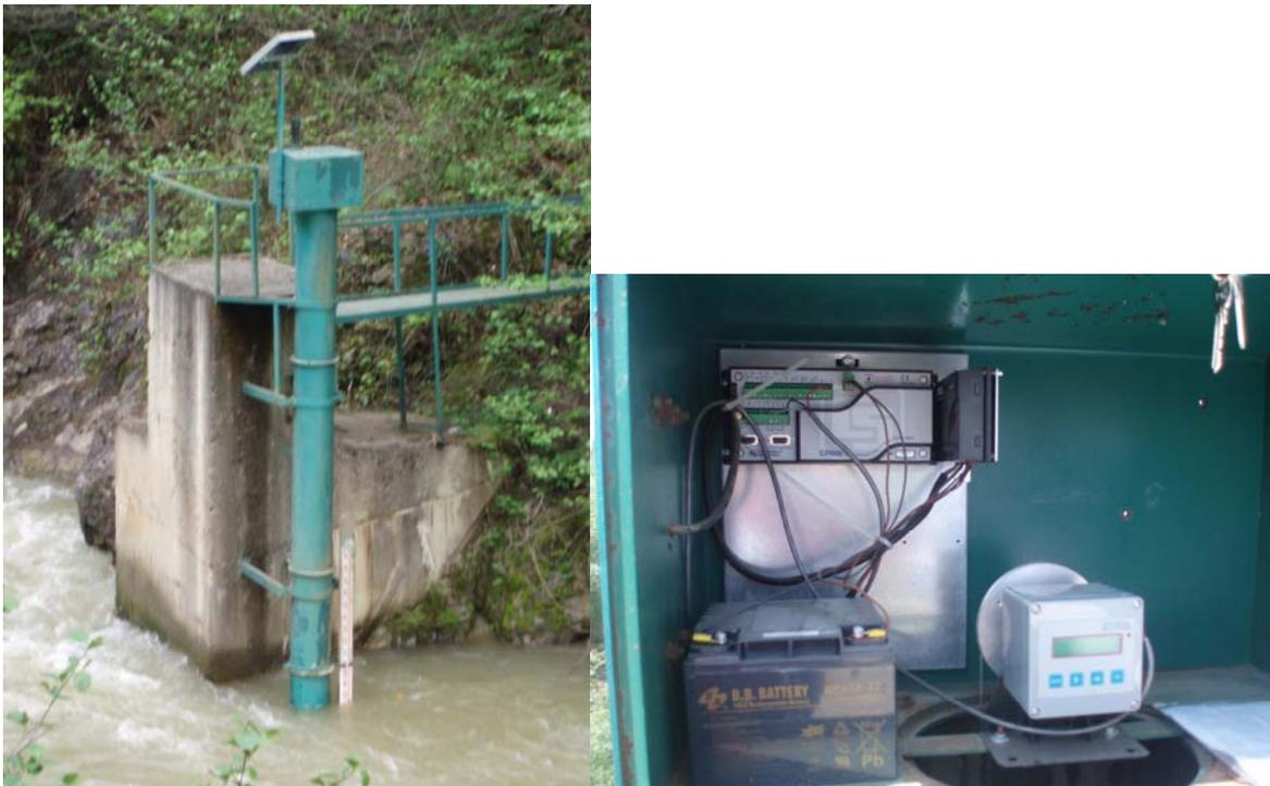
**Figure 5-1: Shaft Encoder installation (left) and shaft encoder, battery and datalogger inside enclosure (right)**
