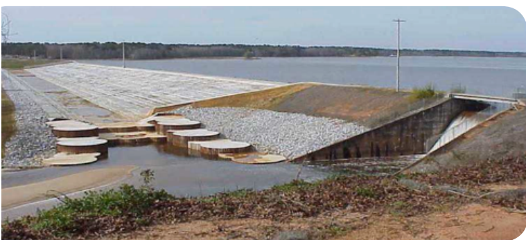
Figure 9.3 7: A view of principal and auxiliary spillways at lake tholocco dam
