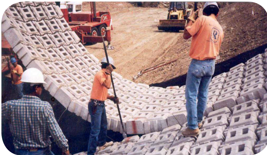
Figure 9.3 2: Installation of the articulated concrete blocks in a channel
