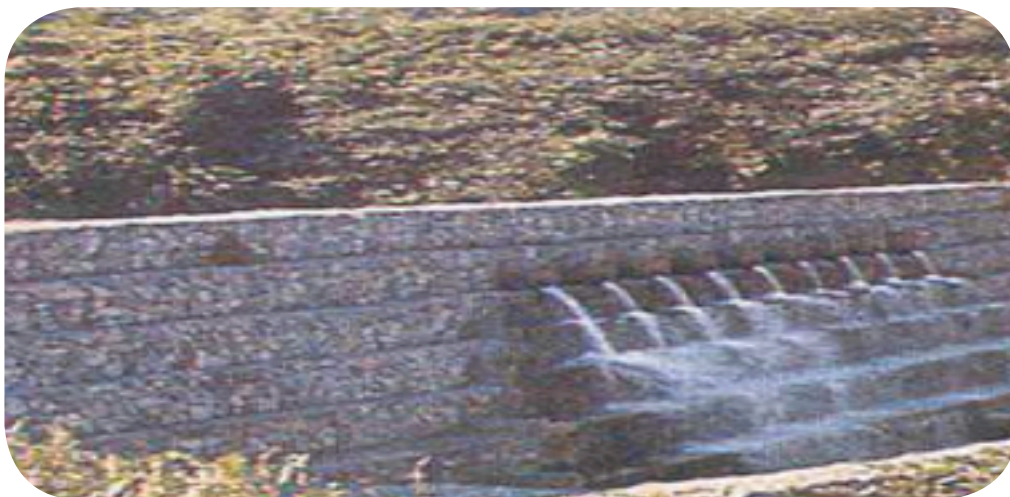
FIGURE 3.5 9: GABION DAM 12 M HIGH - BRAZIL
