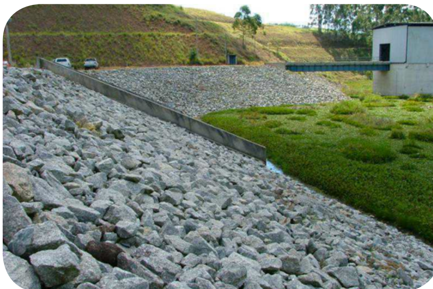
Figure 7.10 2: Upstream gneiss rip-rap at the paraitinga dam, in brazil.
