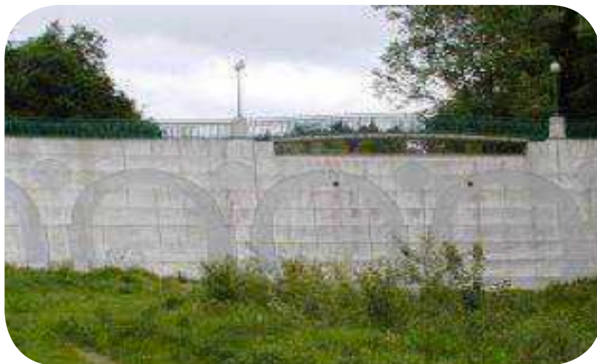
FIGURE 3.5 6: HLINKY CONCRETE GRAVITY DAM, HEIGHT 11M, CZECH REPUBLIC
