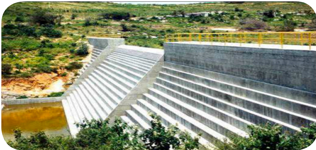
FIGURE 3.5 7: TRAIRAS RCC CONCRETE DAM – BRAZIL
