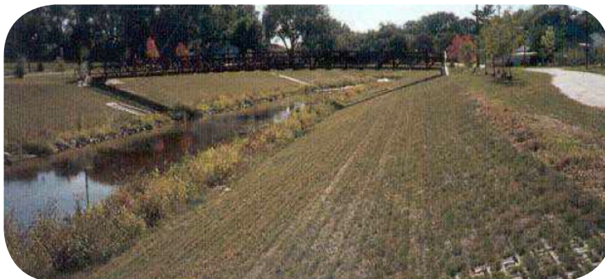
Figure 9.3 3: Lateral slopes protected with concrete blocks and grass
