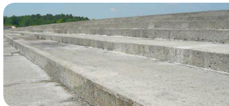
Figure 9.3 8: Excellent condition of rcc steps at tholocco lake dam (Abdo and adaska/07)
