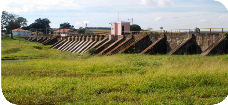
FIGURE 3.5 8: BARRA BUTTRESS CONCRETE DAM, BRAZIL.
