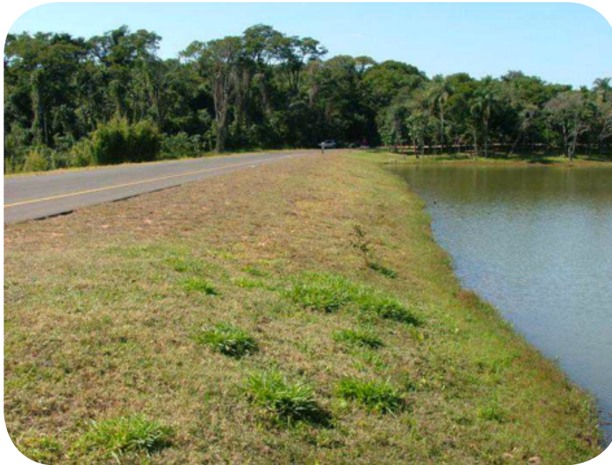
Figure 7.10 3: Upstream slope protection with grass at the chibarro dam, 12 m high, in brazil (fetch = 300 m).
