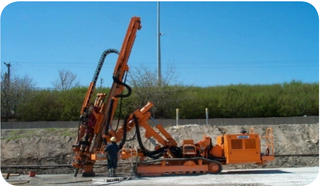
Figure 9.3 12: Grout holes are drilled at optimized angles for rock joints patterns (image from www.Advancedconstructiontechniques.Com/ ).
