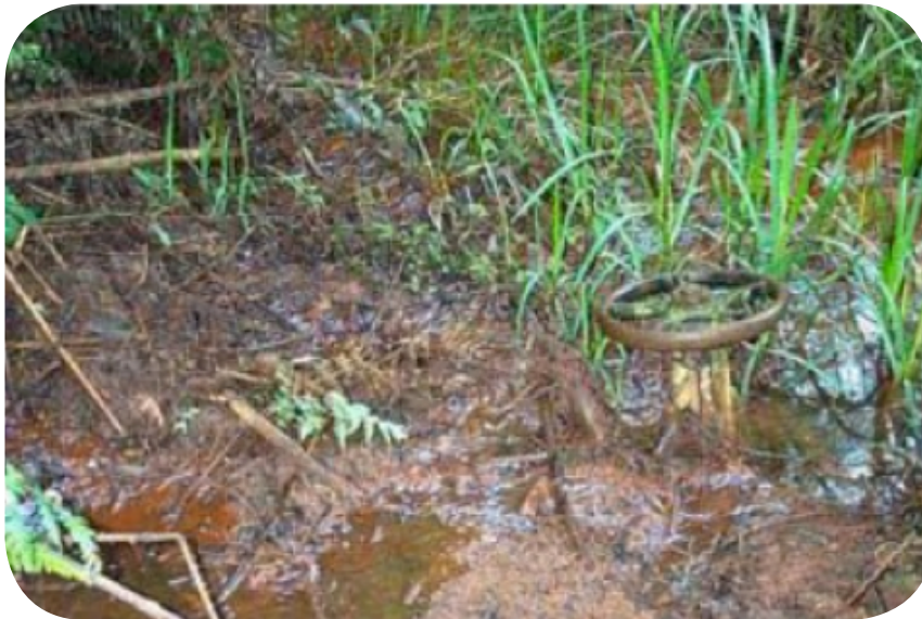
Figure 9.3 18: What are the chances that this valve will work in an emergency? (Smec/2006)
