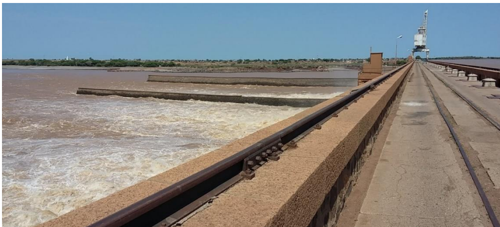
Figure 23: Sennar Dam at Blue Nile, view downstream
