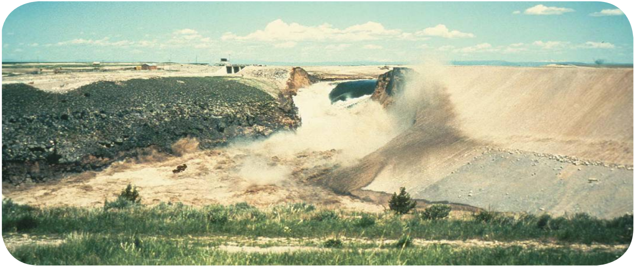
Figure 5-1 Teton dam failure
